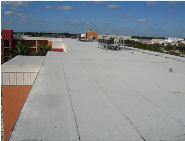
View from roof top looking West.
