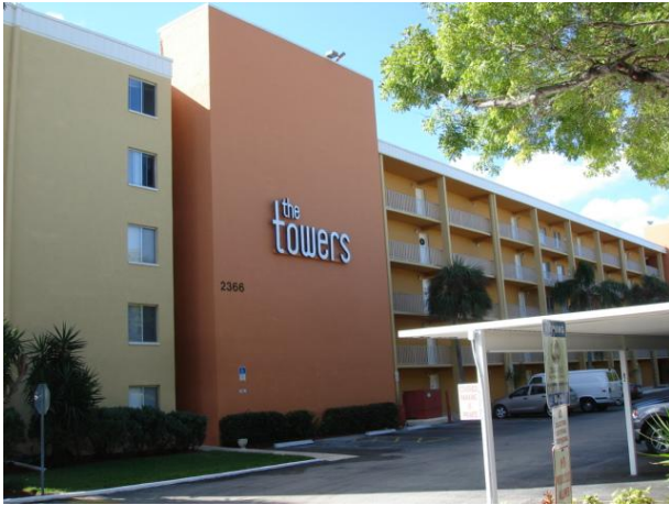
Front elevation of building.
