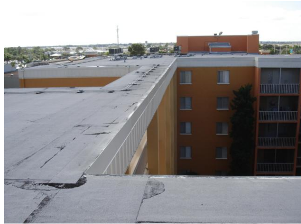
View from roof top looking South.
