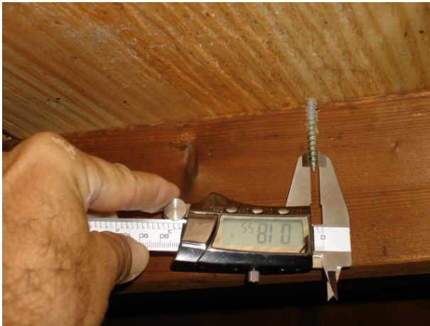
Roof decking fastened with screws (.18").
