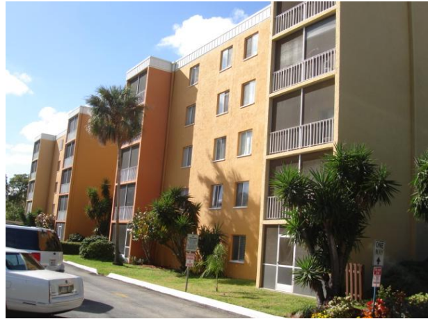
Rear elevation of building.
