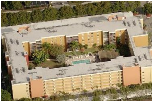
Aerial North view of building.
