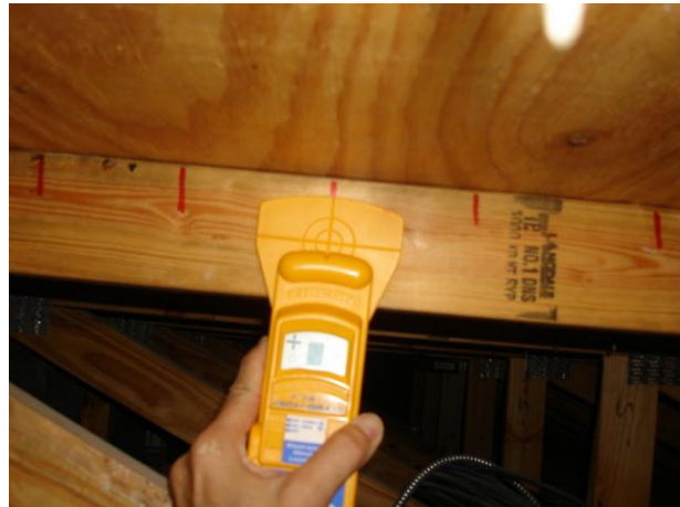
Roof decking attached in a 6/6 pattern.
