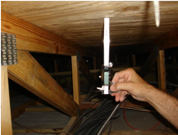
Roof decking is measured as 15/32" plywood.
