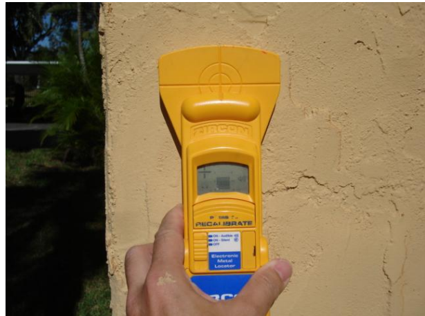
Exterior walls are reinforced masonry.
