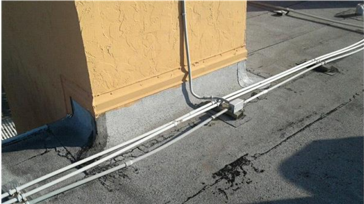
004F - Base Flashings
