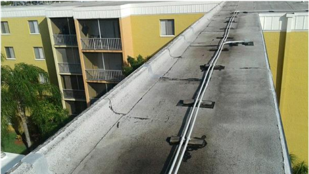
004F - Base Flashings
