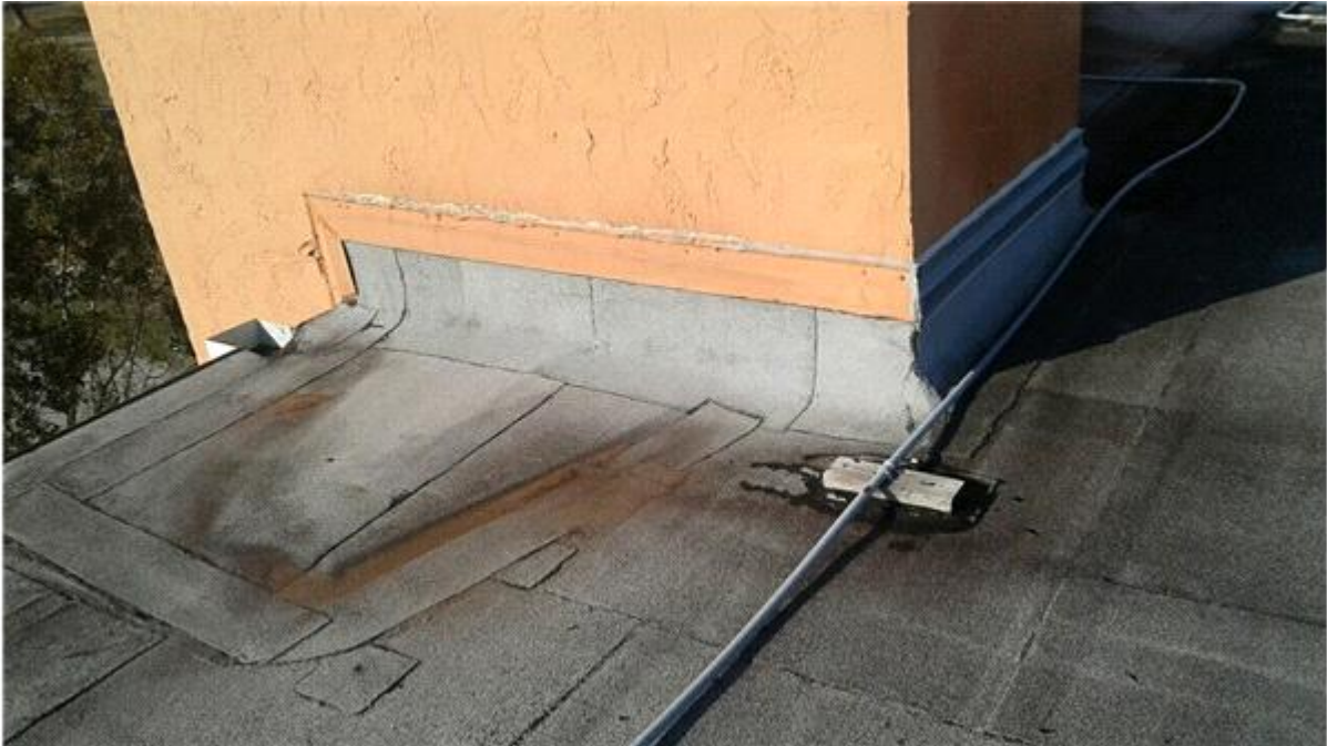
004F - Base Flashings
