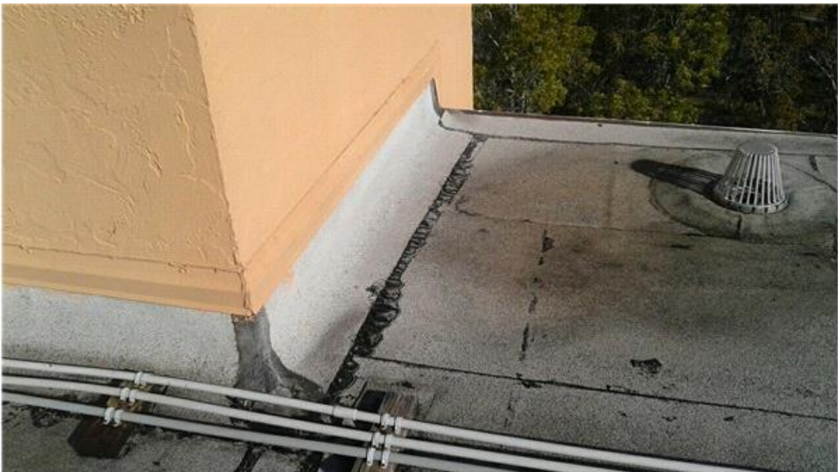
004F - Base Flashings
