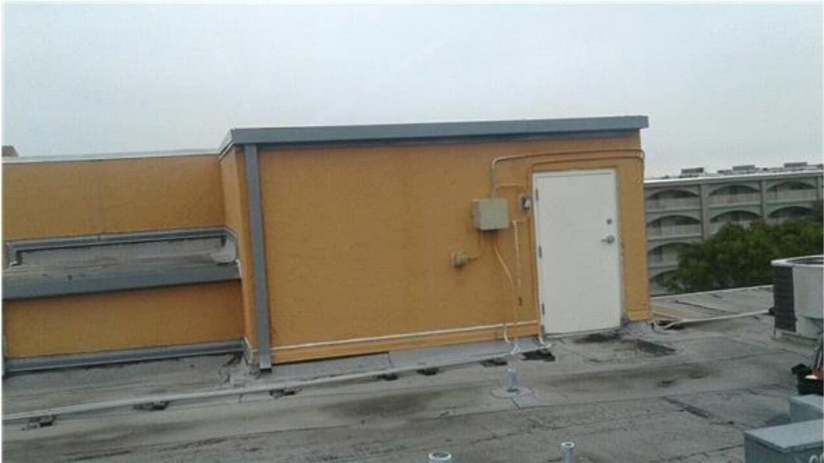
Stairwell Roof Building Identification
