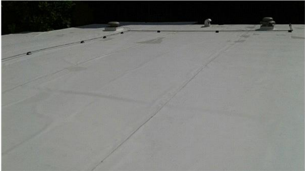
029- Roof overview General roof overview
