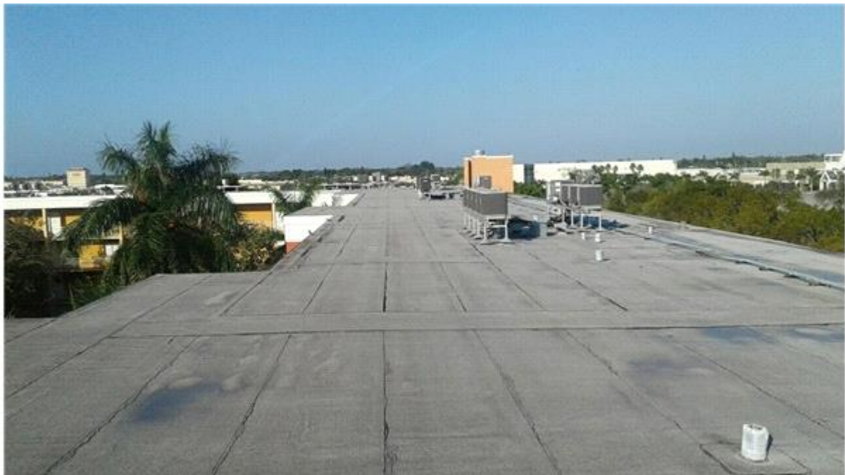
029- Roof overview General roof overview
