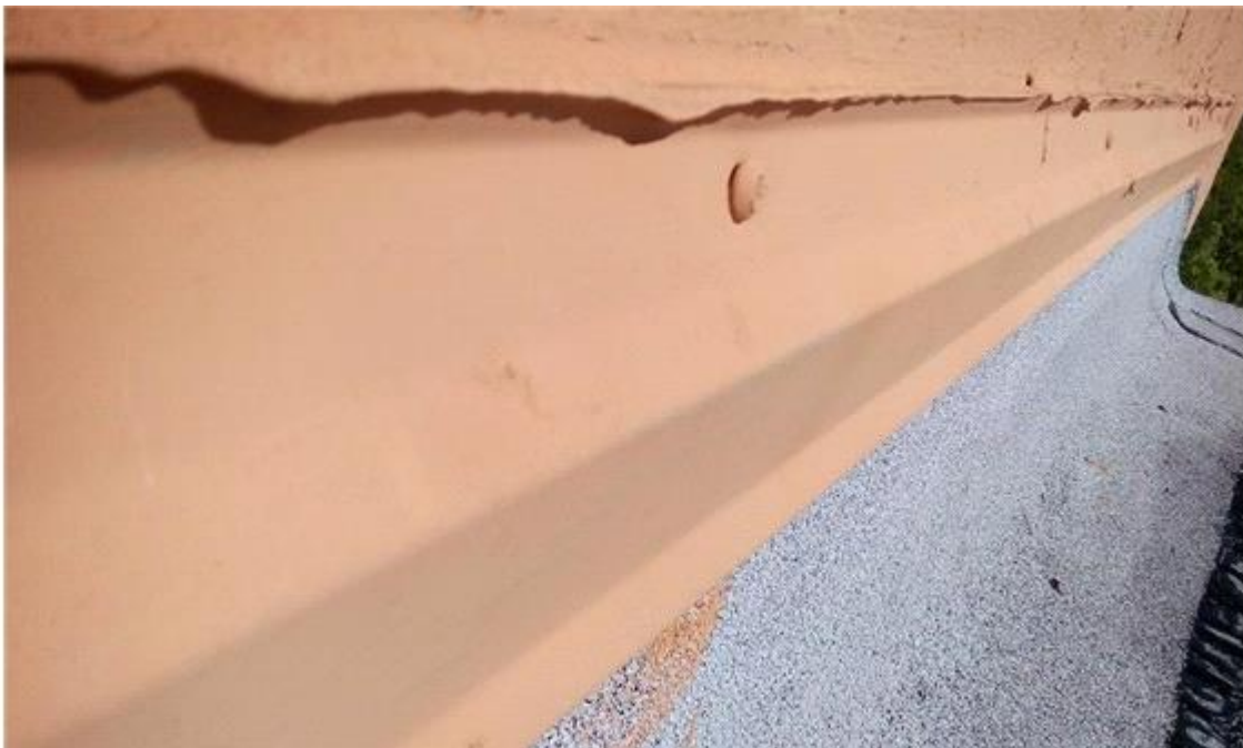
005G- Counter Flashings
