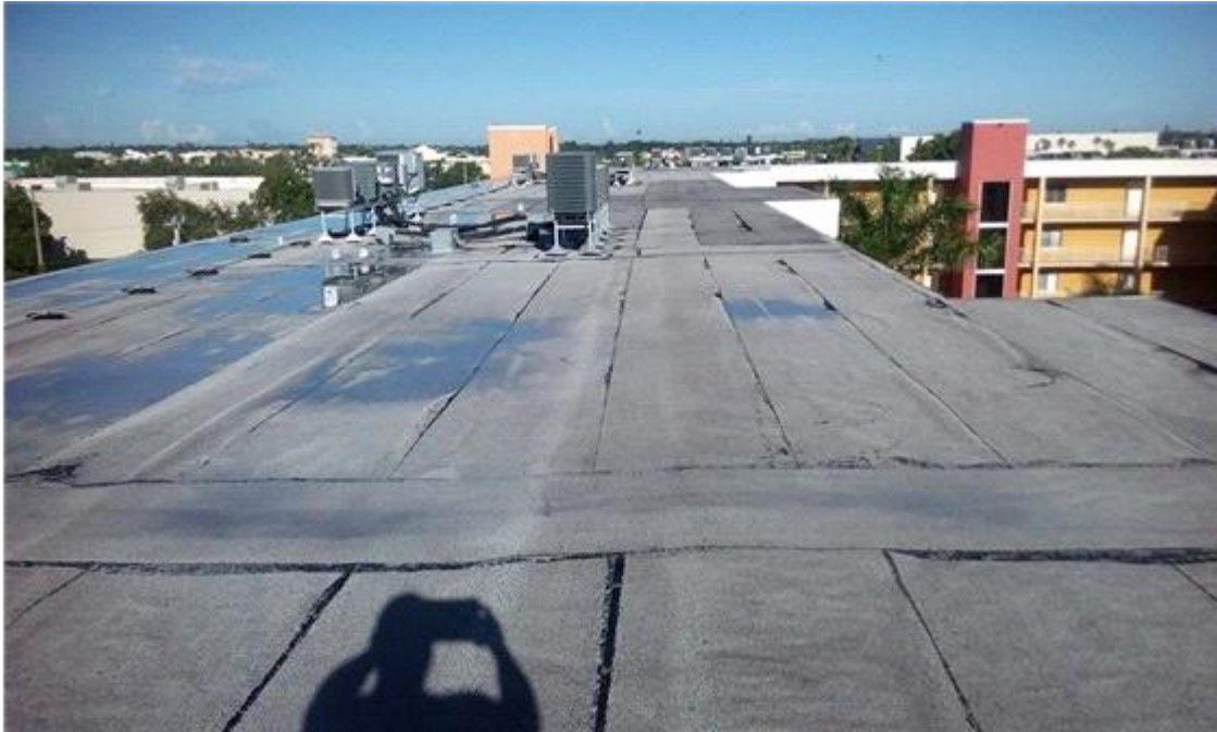
002F - Appearance Overview
