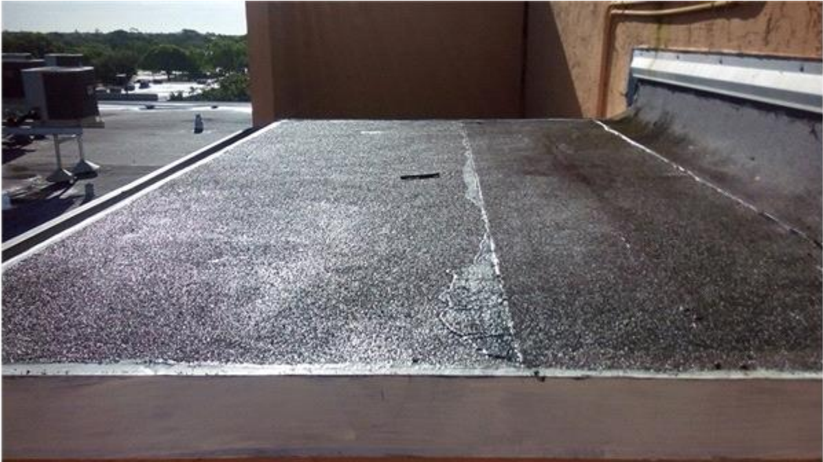
001F - Surface Overview
