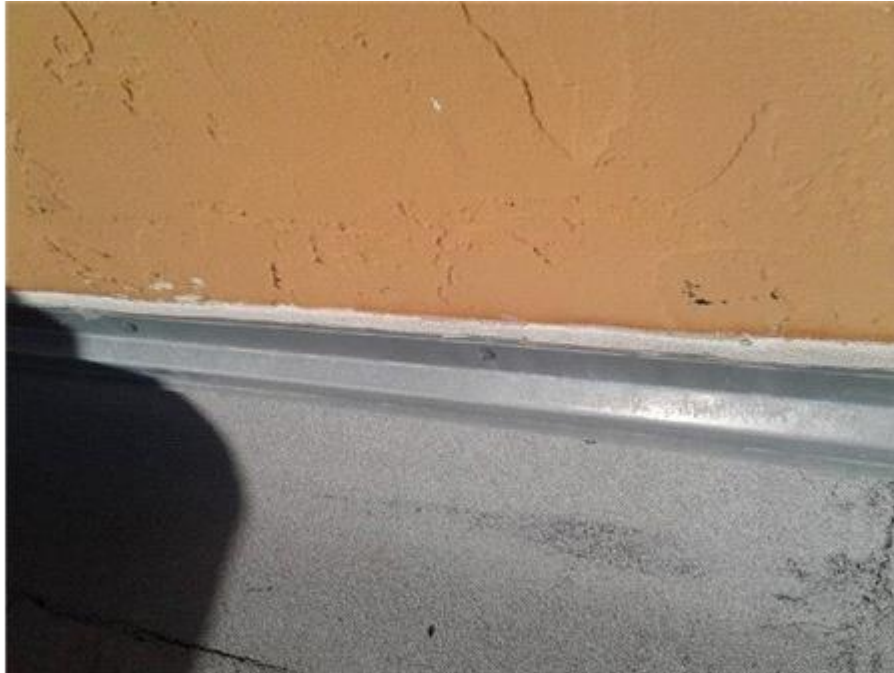
Sealant Deterioration/Failure
