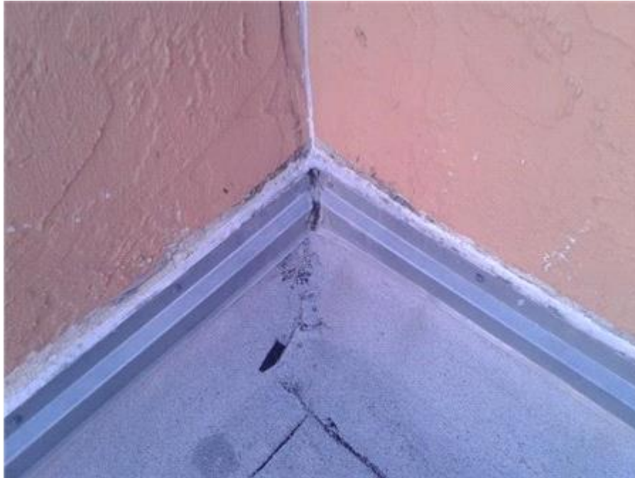
Sealant Deterioration/Failure
