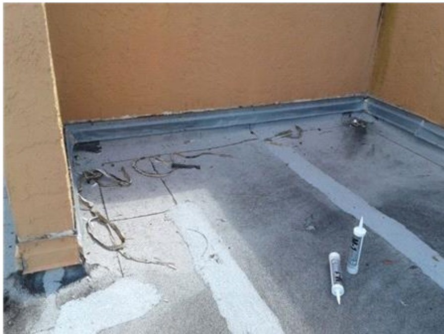
028- Sealant Deterioration/Failure
