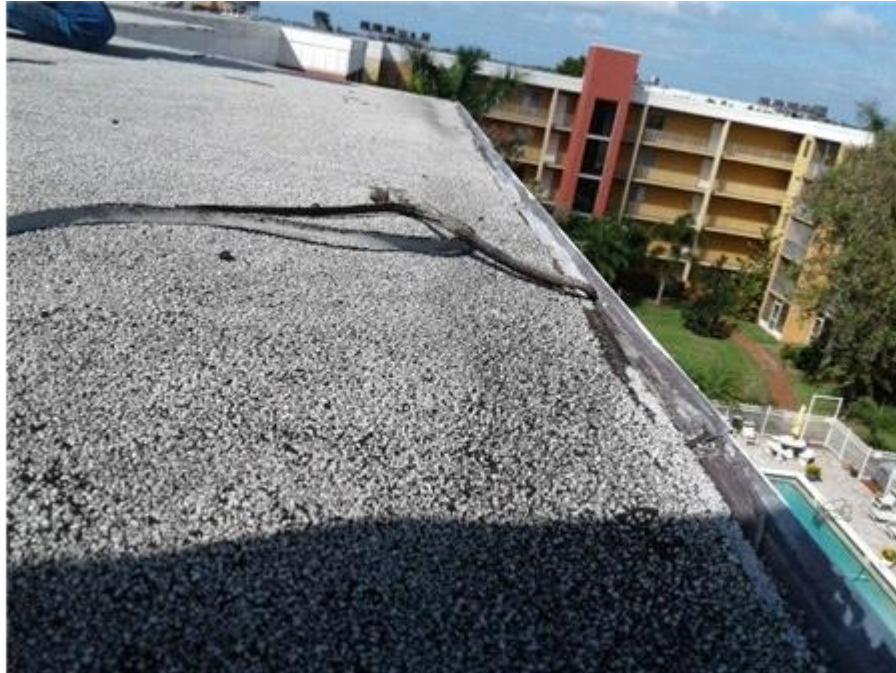
028- Sealant Deterioration/Failure
