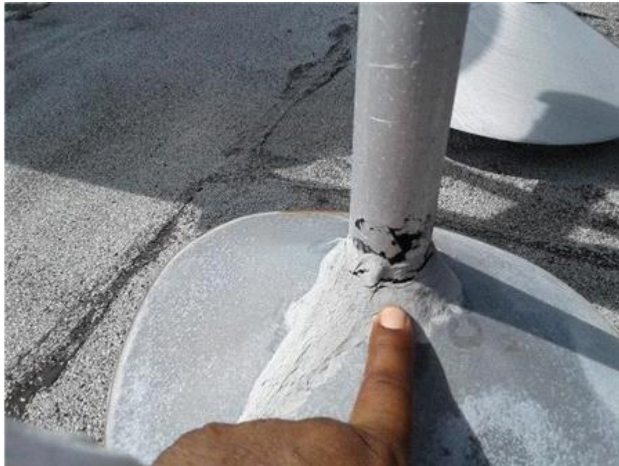
014-Sealant Failure
