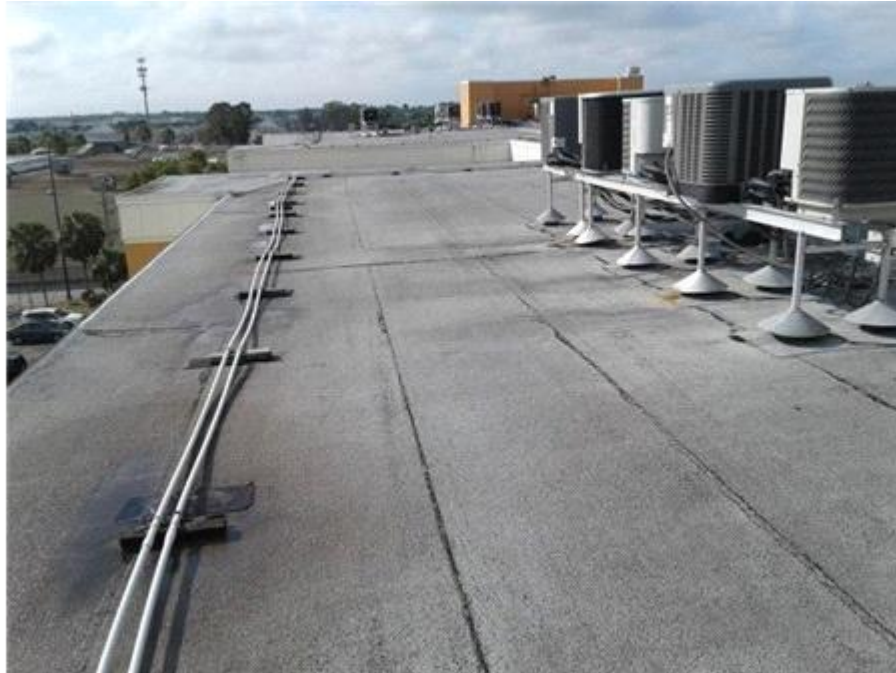
029- Roof Overview General roof overview
