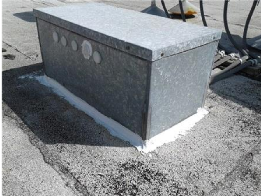
015-Sealant Repair
