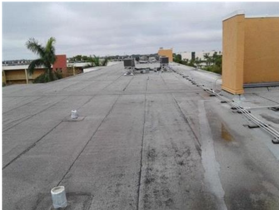
001G- The Towers - Main Roof
