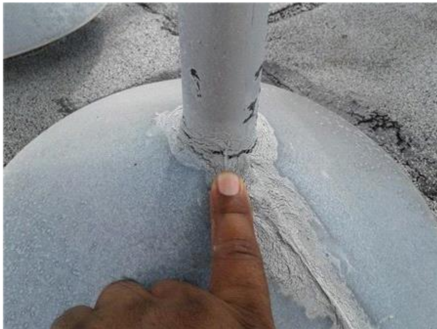
014-Sealant Failure
