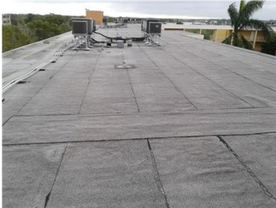
029- Roof Overview General roof overview
