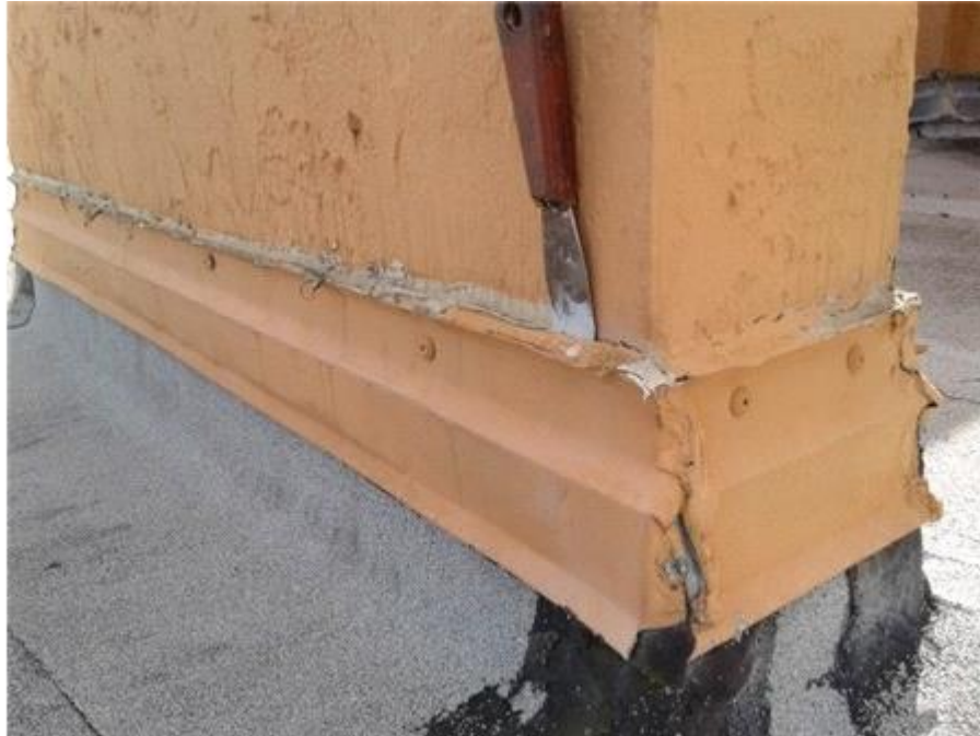
028- Sealant Deterioration/Failure
