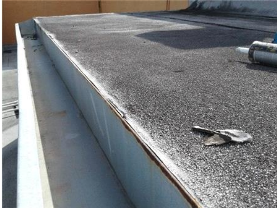
028- Sealant Deterioration/Failure
