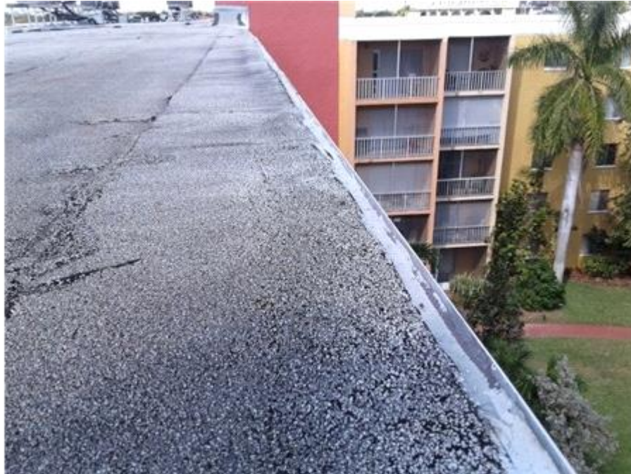
028- Sealant Deterioration/Failure
