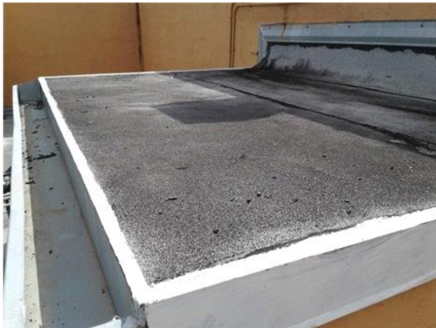
015-Sealant Repair
