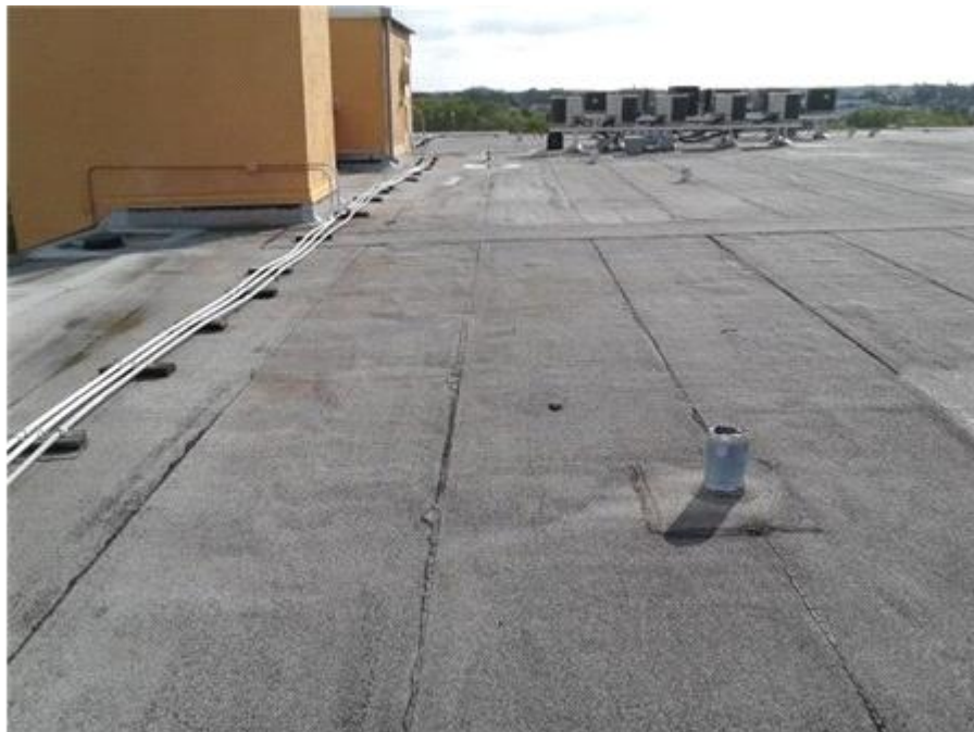
029- Roof Overview General roof overview
