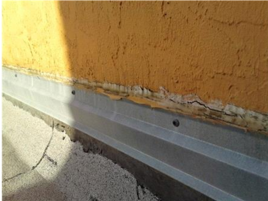
028- Sealant Deterioration/Failure
