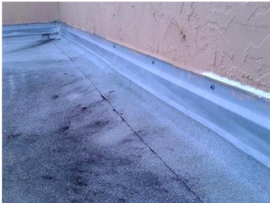
005G- Counter Flashing
