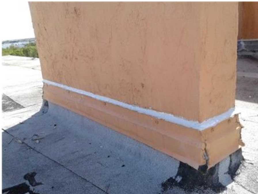
015-Sealant Repair
