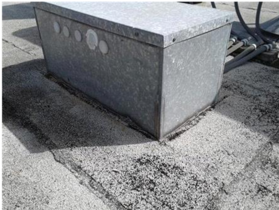
014-Sealant Failure
