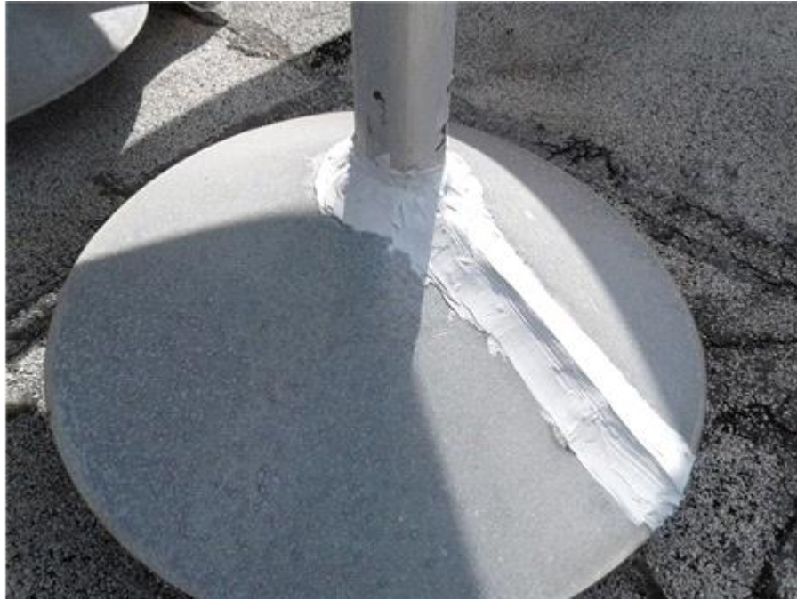
015-Sealant Repair
