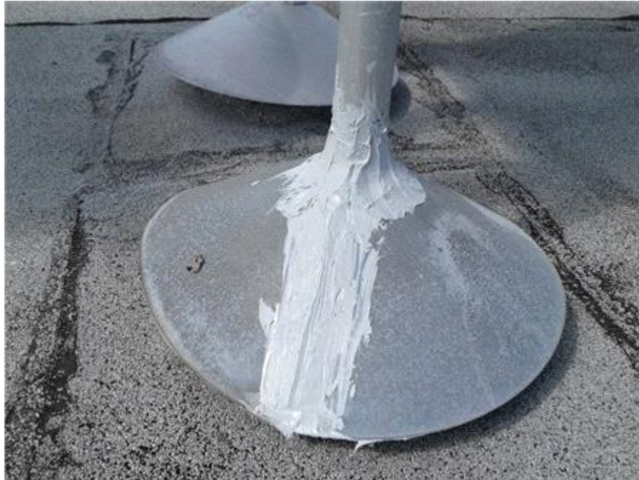
015-Sealant Repair
