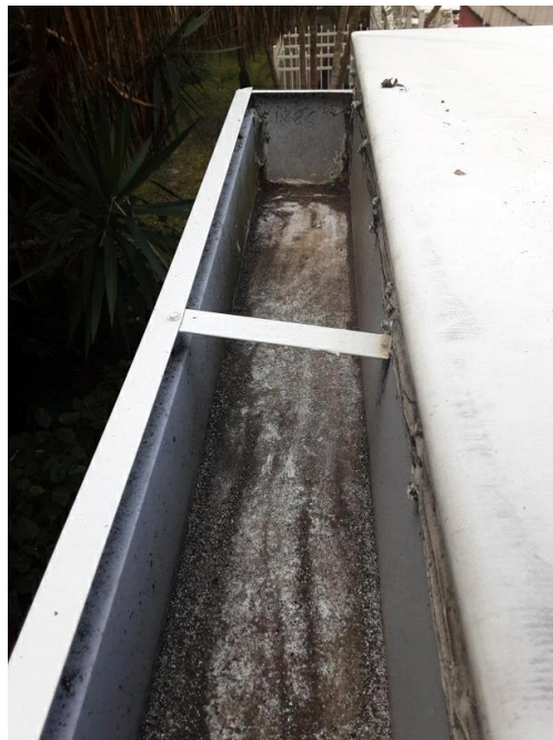
Removed Debris from Gutters
