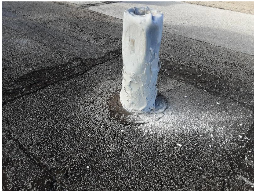
Lead Boot-Temporary Repair
