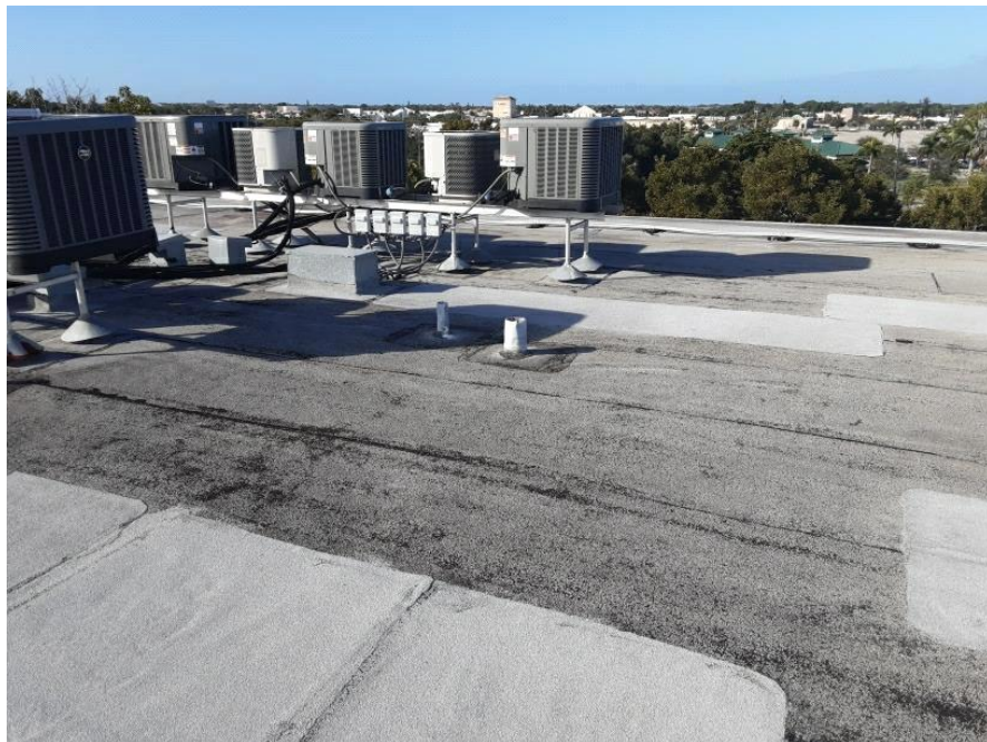
Lead Boot-Damaged
