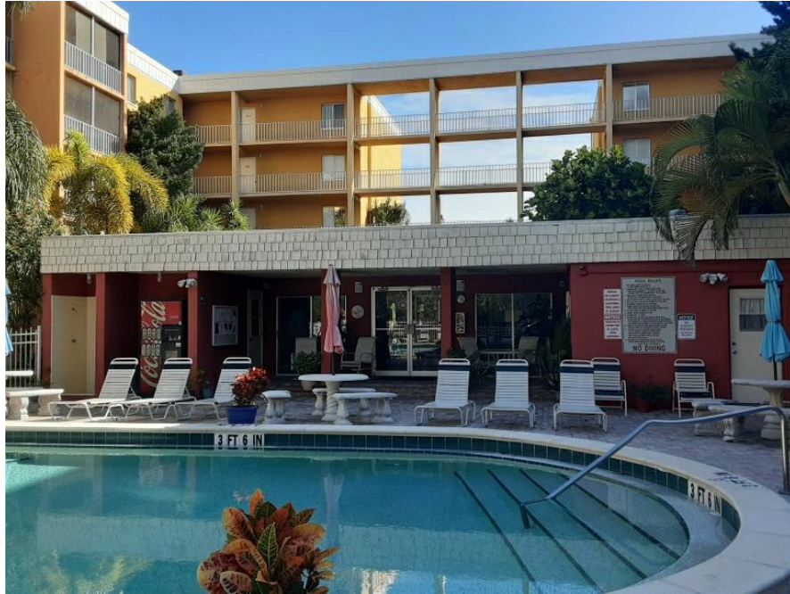
Pool House Building Identification
