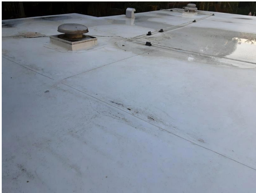
Membrane Overview The membrane appears to be in good, maintainable condition.
