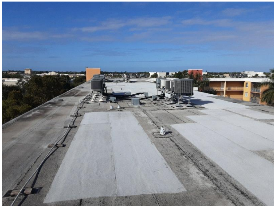
Roof Overview General roof overview.
