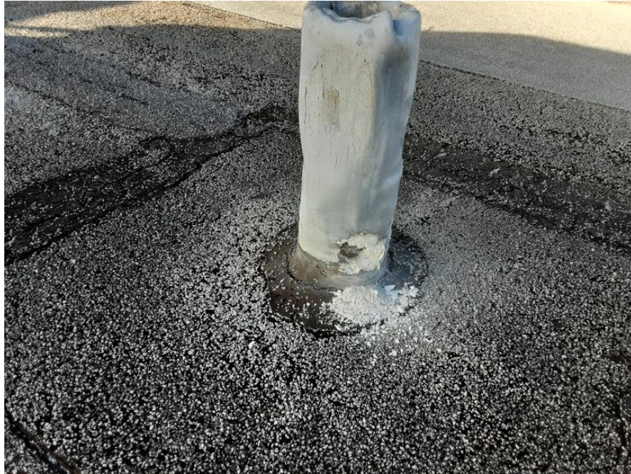
Lead Boot-Damaged
