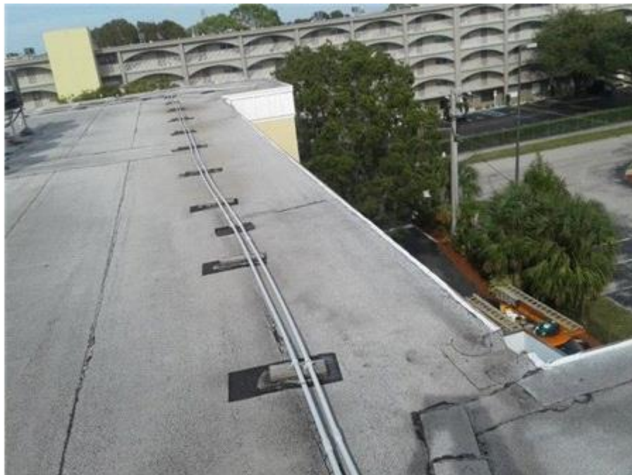
Elevator Shaft Roof: Roof Edge
