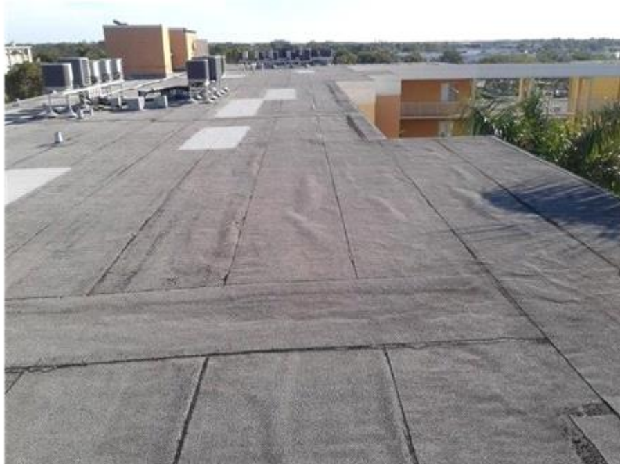
Main Roof: Roof Overview
