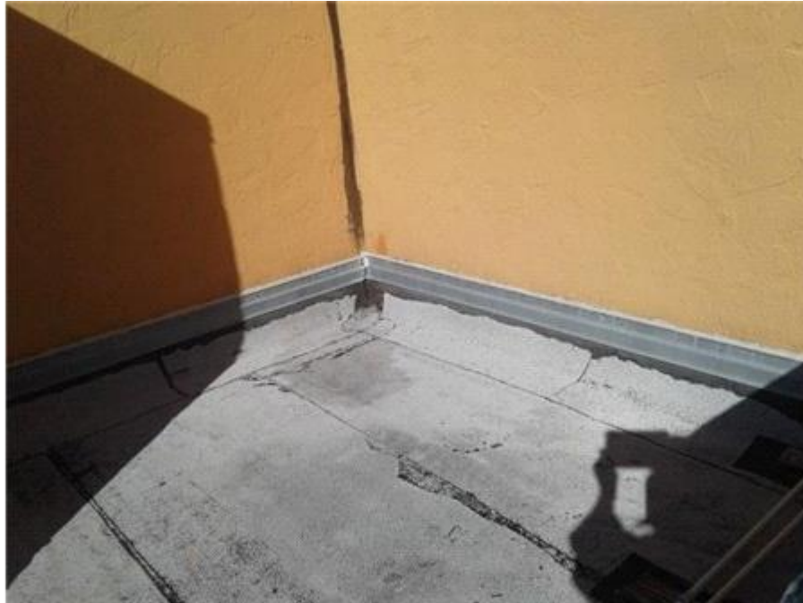
Main Roof: Counter Flashings
