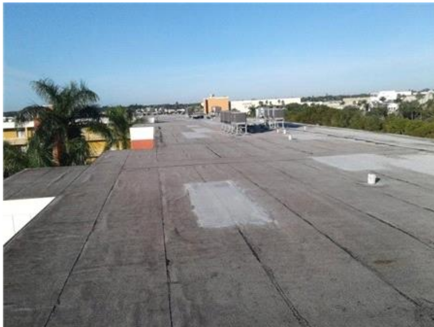
Main Roof: Roof Overview General roof overview
