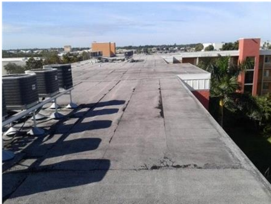
Elevator Shaft Roof: Surface Overview
