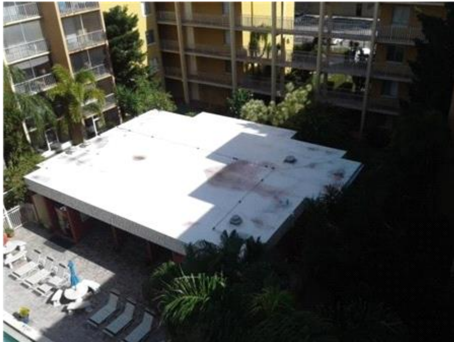
Clubhouse: Roof Overview
