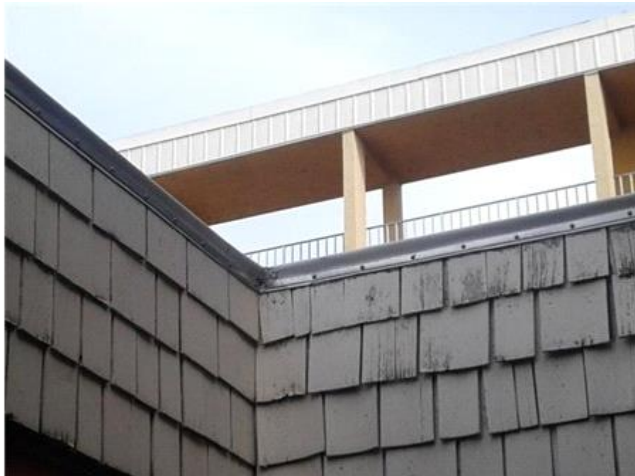
Clubhouse: Roof Edge
