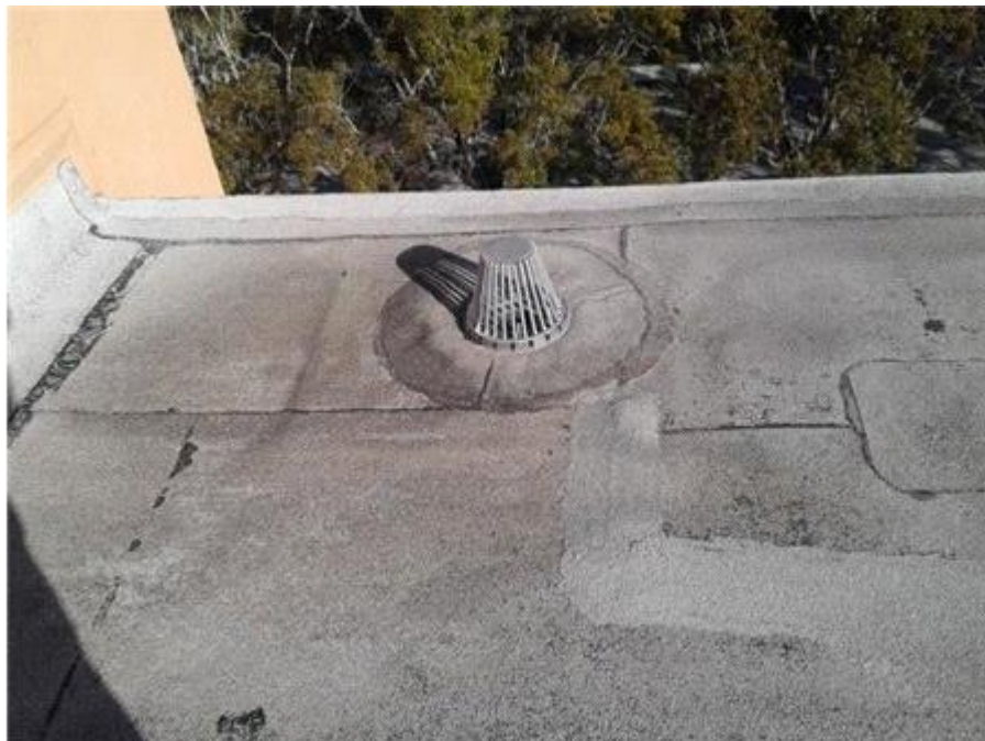
Main Roof: Roof Drains
