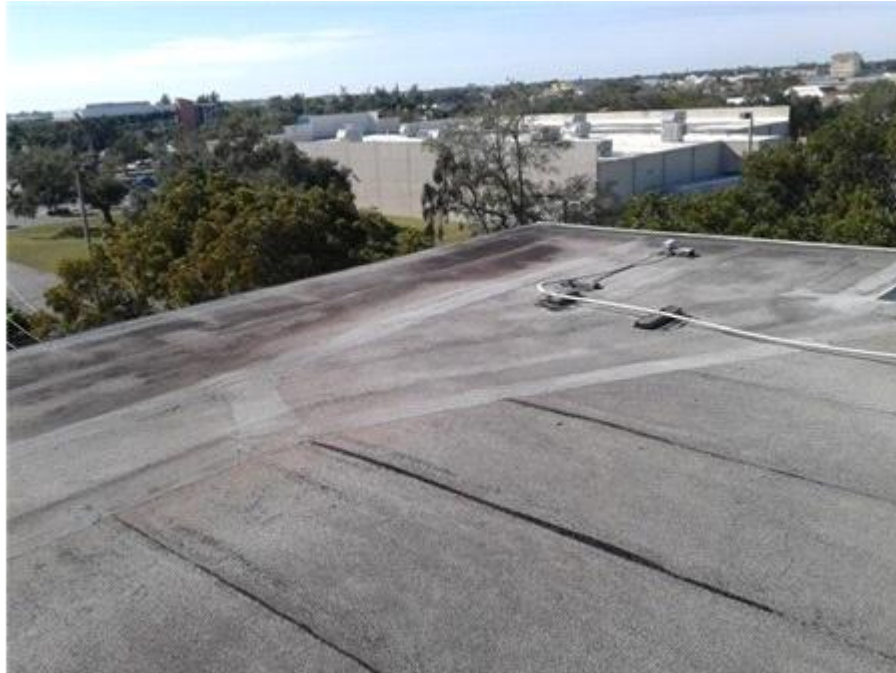
Elevator Shaft Roof: Surface Overview
