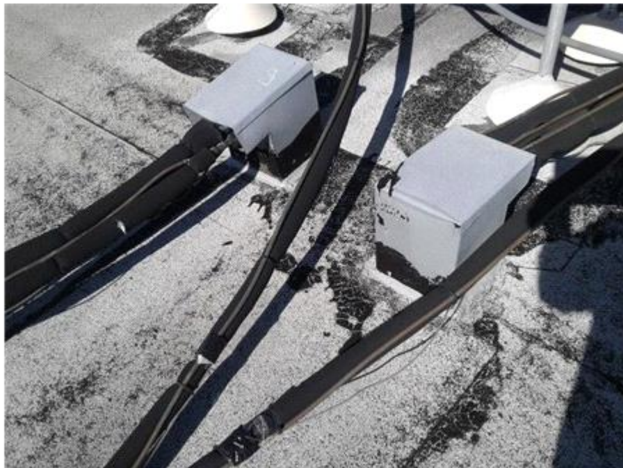
Elevator Shaft Roof: Sealant Repair
