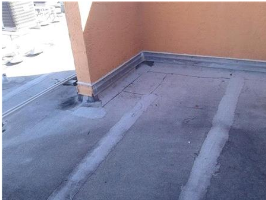
Stairwell Roof: Removed Debris on Roof
