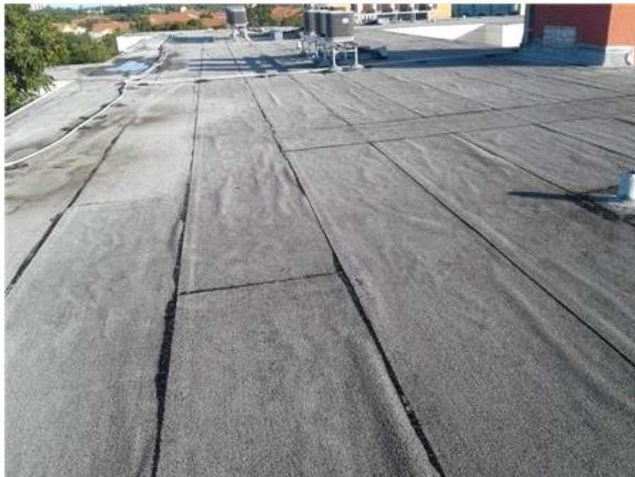
Main Roof: Membrane Overview
