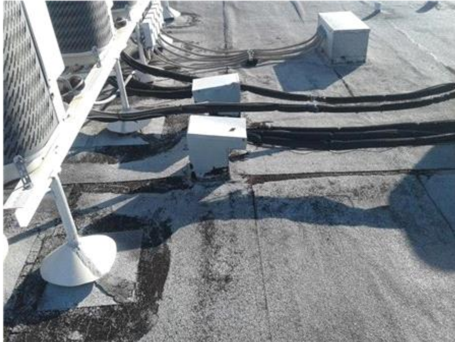
Main Roof: Equipment Housing
