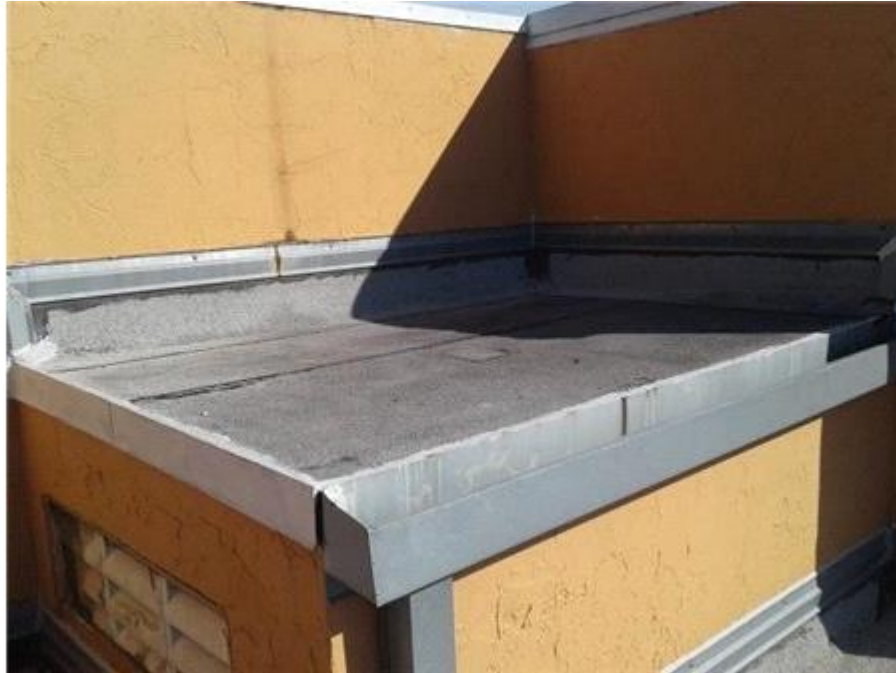
Stairwell Roof: Appearance Overview
