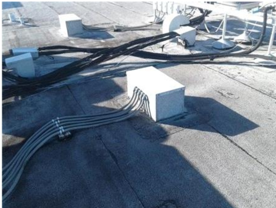
Main Roof: Equipment Housing
