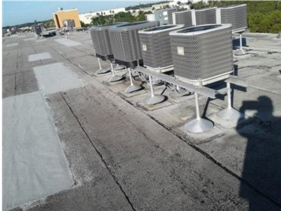
Main Roof: Appearance Overview
