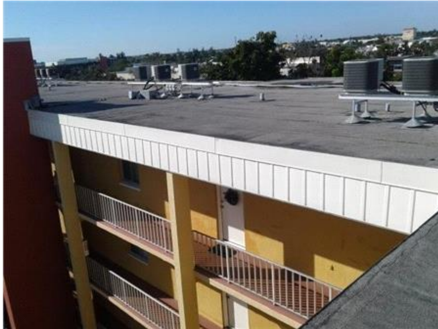
Main Roof: Edge Metal
