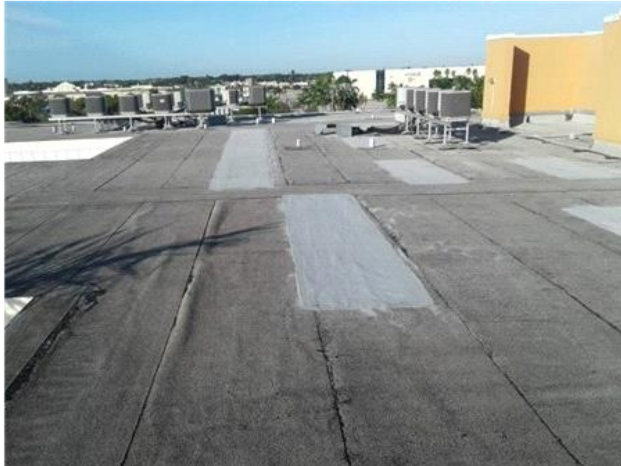
Main Roof: Surface Overview
