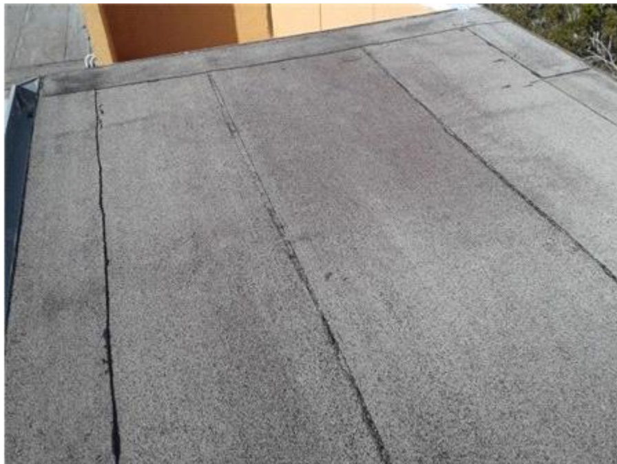
Stairwell Roof: Base Flashings
