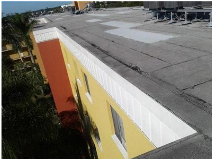
Main Roof: Edge Metal
