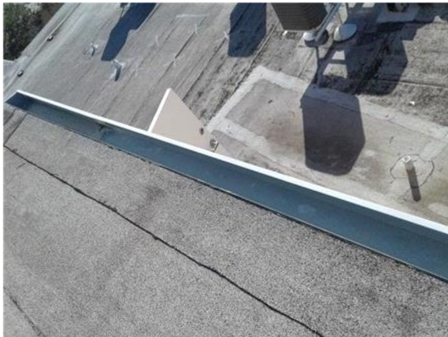
Stairwell Roof: Gutter Metal
