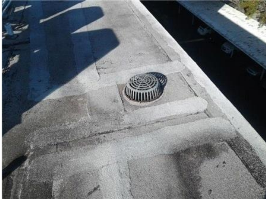
Main Roof: Roof Drains
