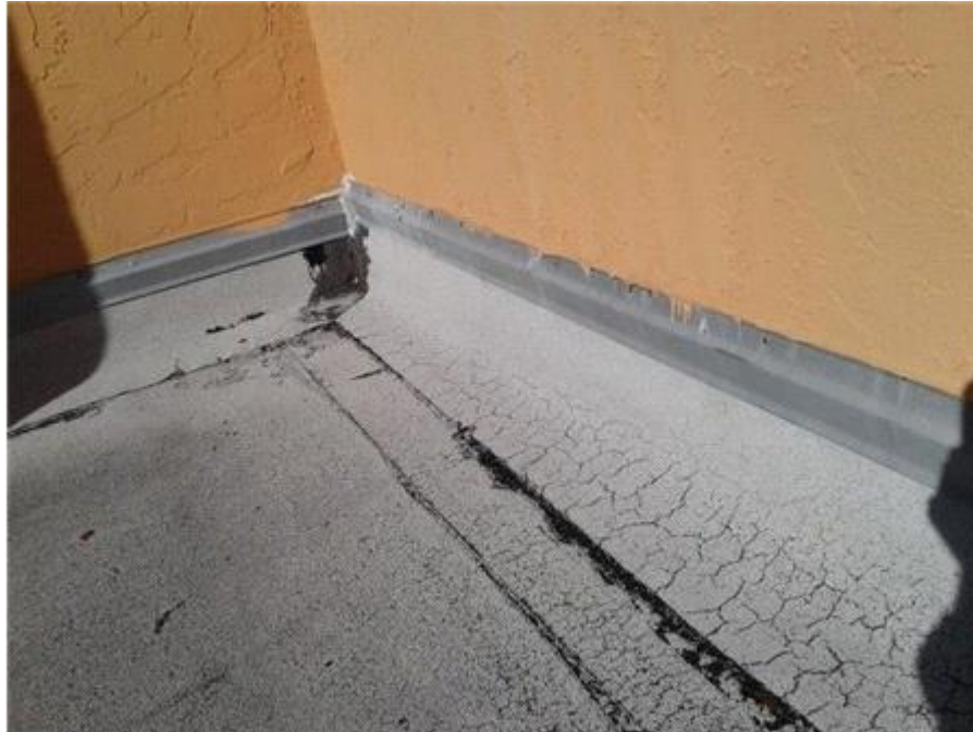
Main Roof: Counter Flashings
