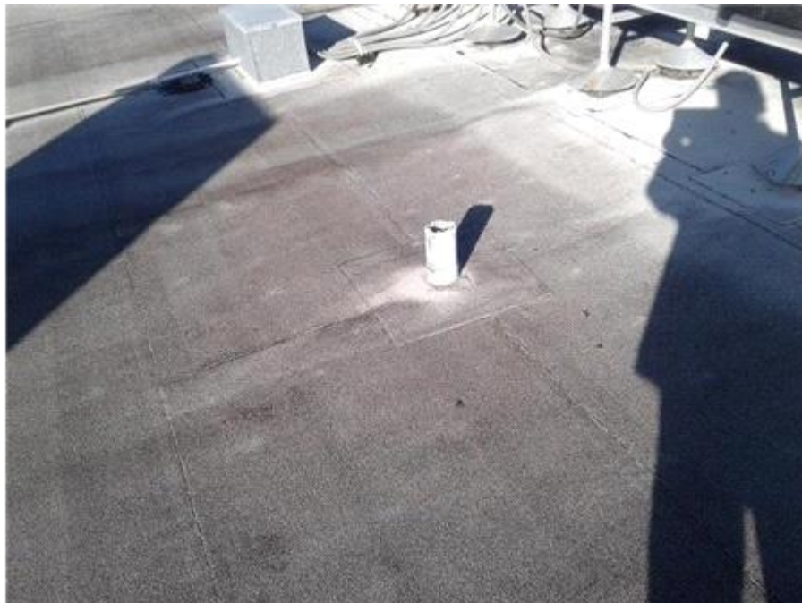
Main Roof: Lead Boots
