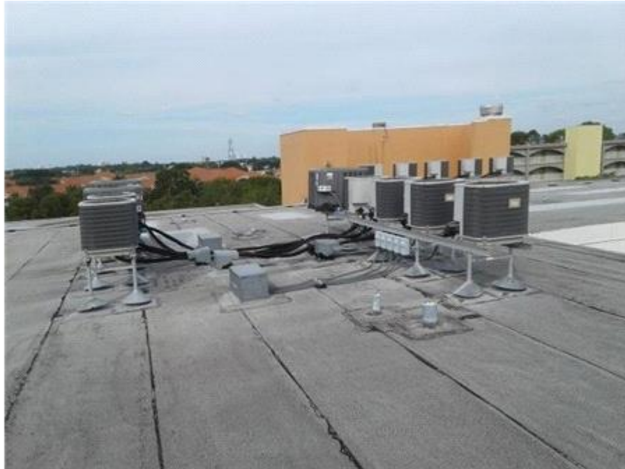
Elevator Shaft Roof: Appearance Overview
