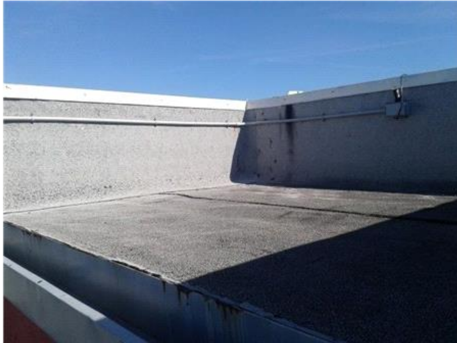
Elevator Shaft Roof: Appearance Overview
