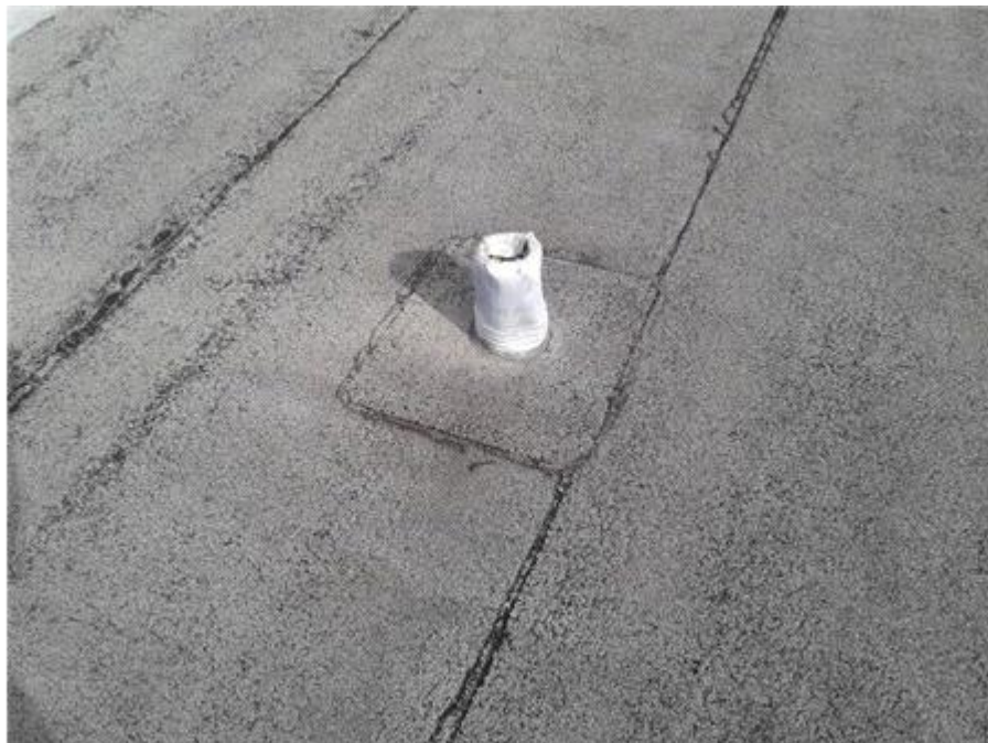
Elevator Shaft Roof: Lead Boots
