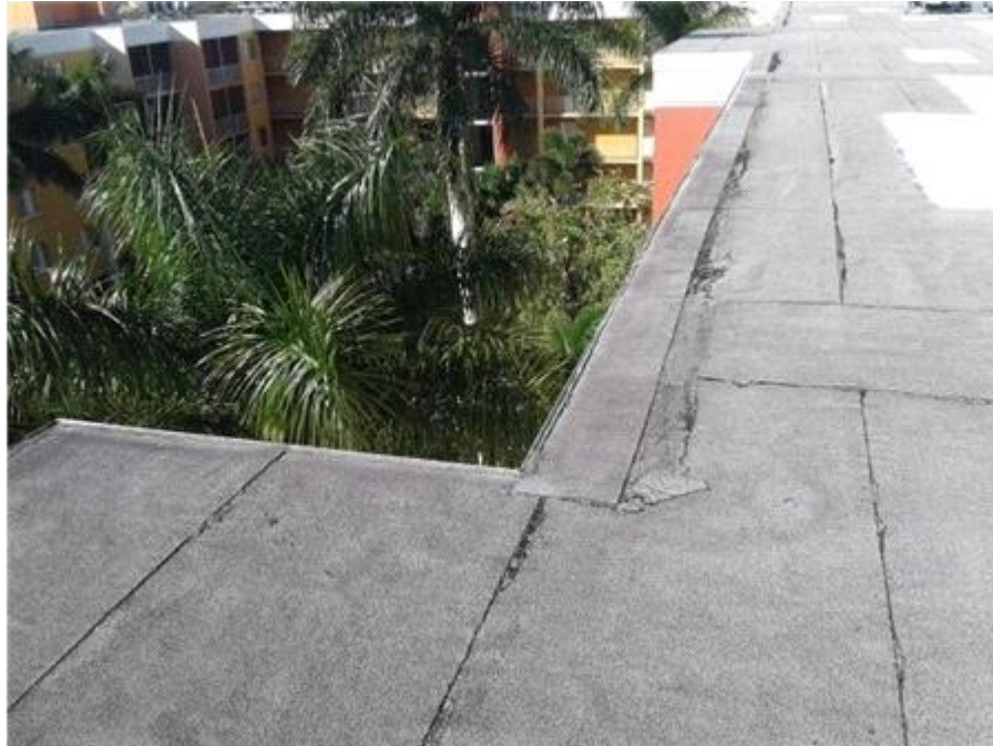
Main Roof: Roof Edge
