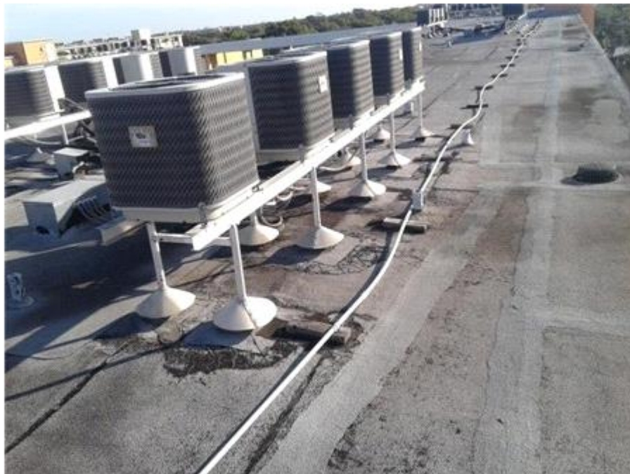
Main Roof: Appearance Overview
