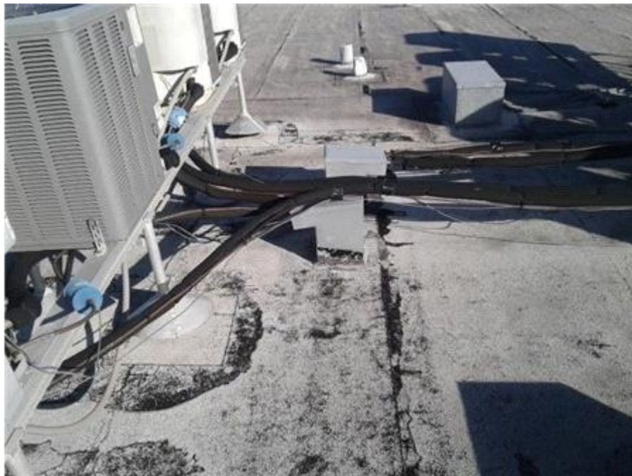
Main Roof: Equipment Housing
