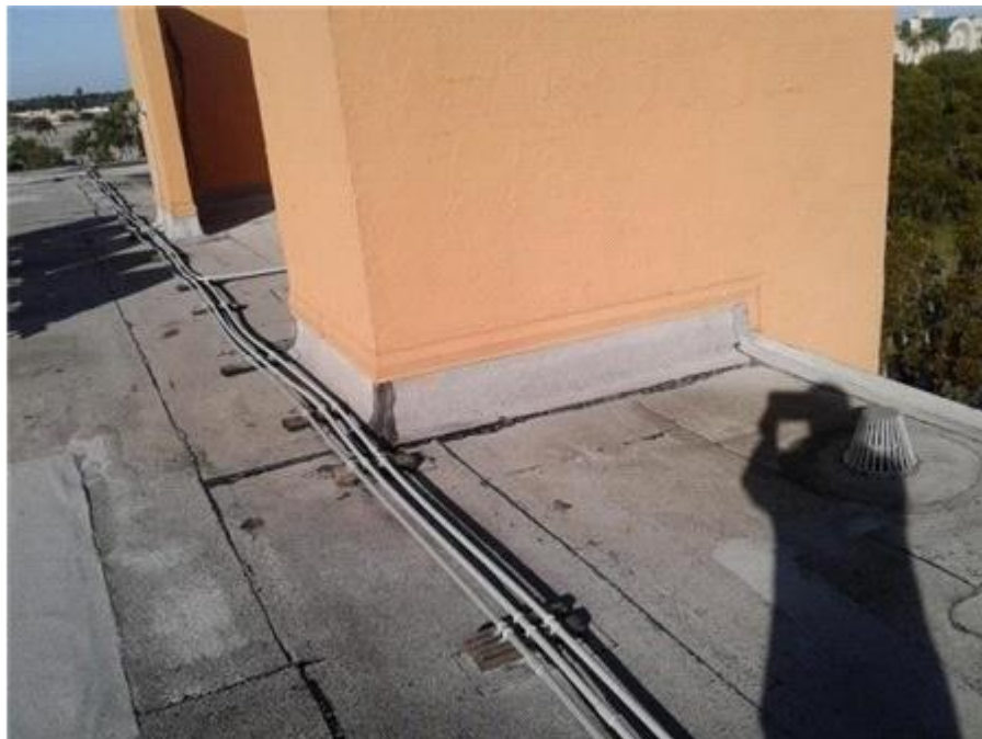
Main Roof: Base Flashings
