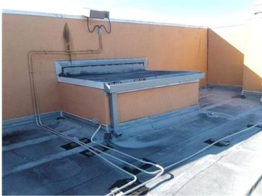
Stairwell Roof: Appearance Overview
