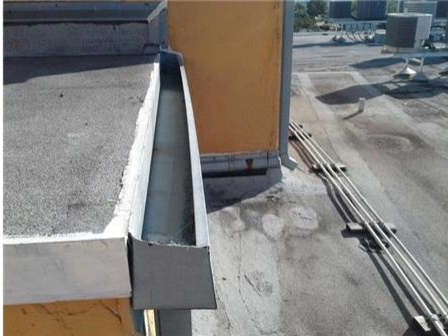
Stairwell Roof: Gutters
