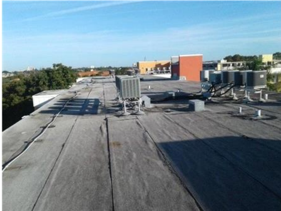
Main Roof: Roof Overview
