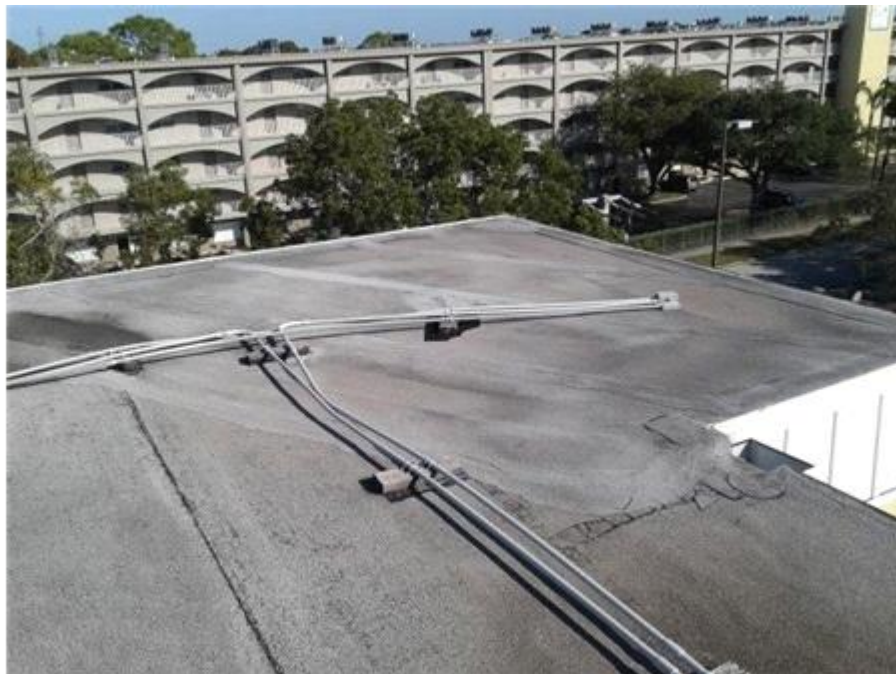
Stairwell Roof: Surface Overview
