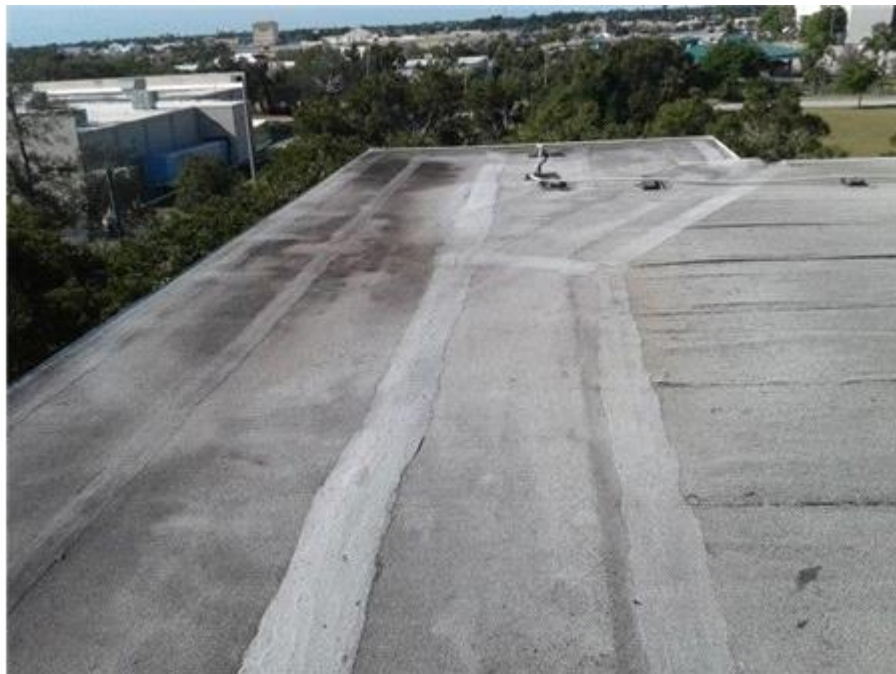
Elevator Shaft Roof: Surface Overview
