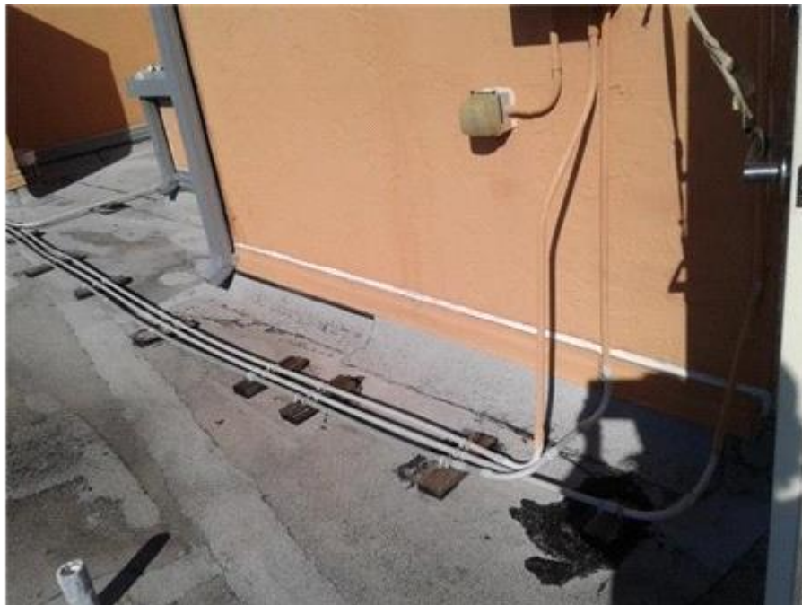
Main Roof: Counter Flashings
