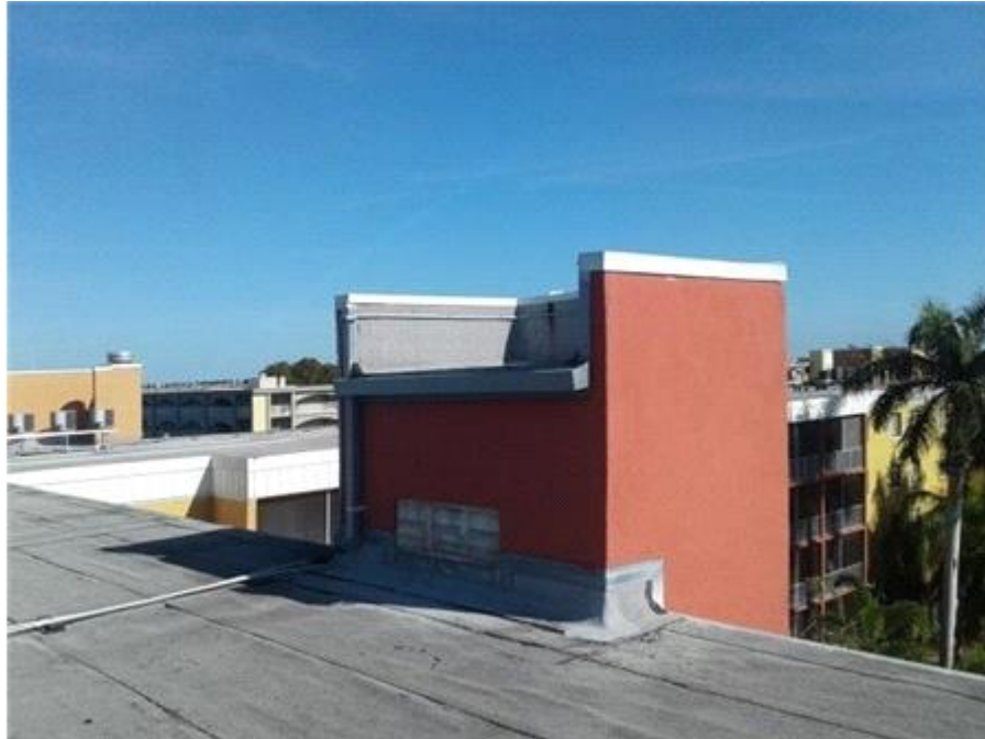
Elevator Shaft Roof Location Identification
