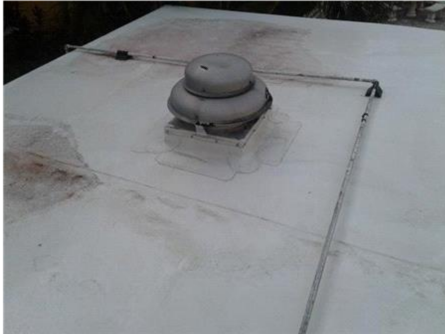
Clubhouse: Roof Vents
