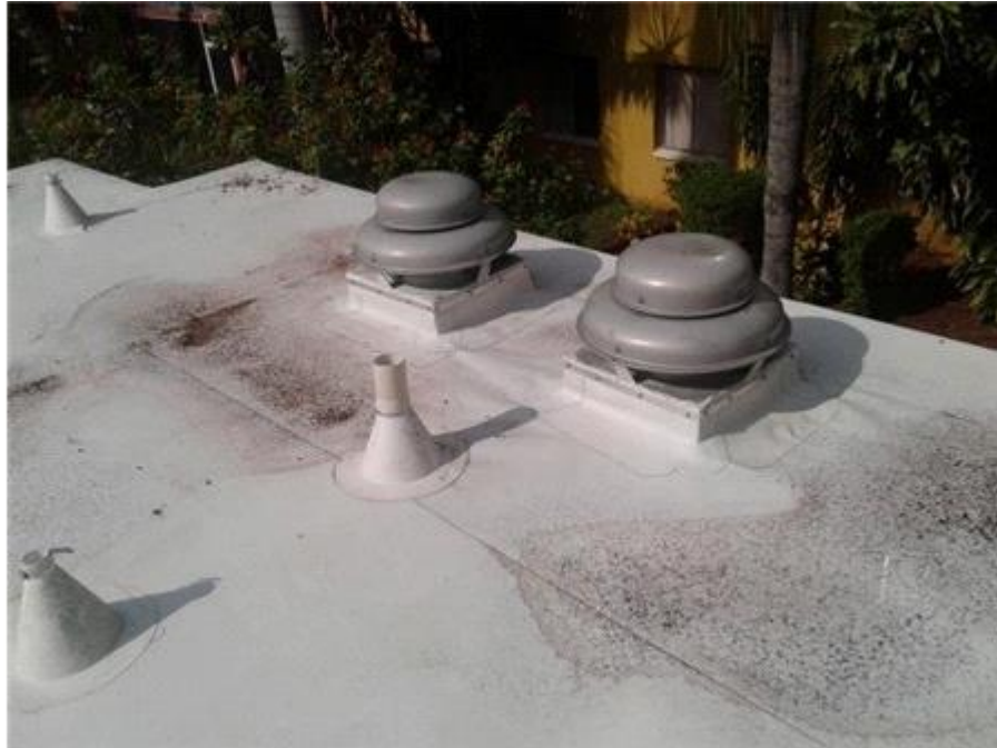
Clubhouse: Base Flashings
