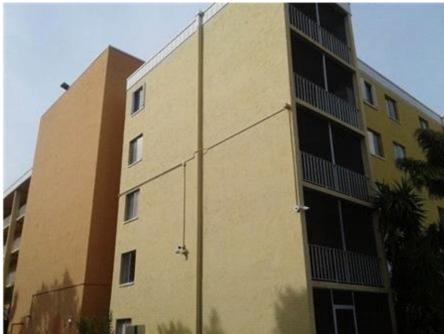
Elevator Shaft Roof: Downspouts
