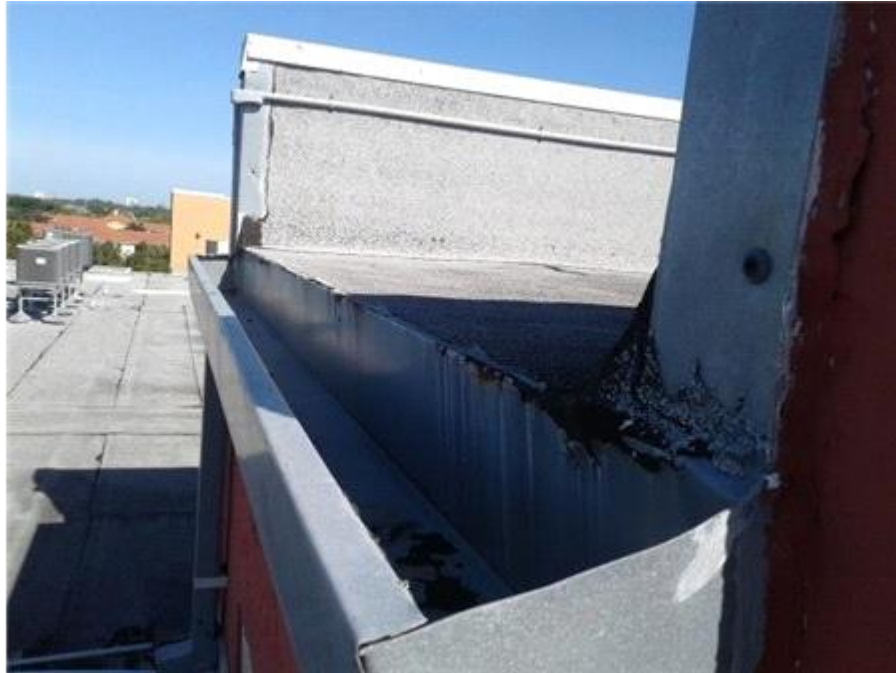
Elevator Shaft Roof: Gutters
