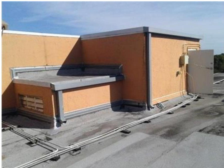
Stairwell Roof: Appearance Overview
