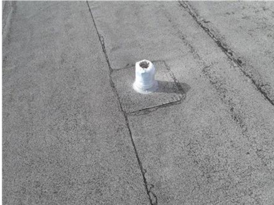
Elevator Shaft Roof: Lead Boots
