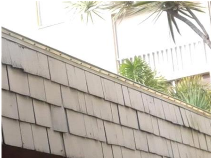
Clubhouse: Roof Edge
