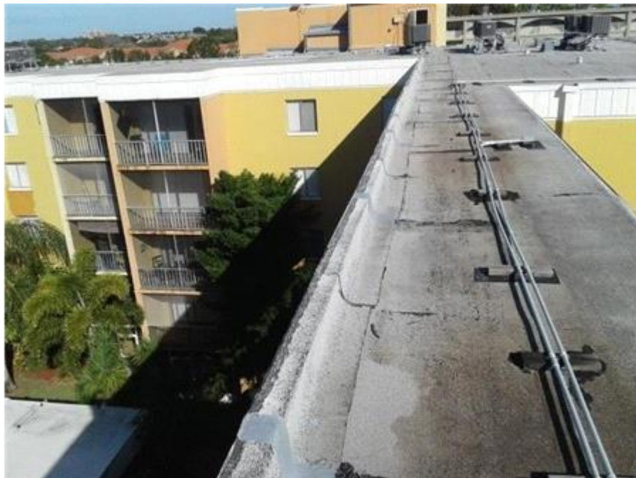
Main Roof: Roof Edge
