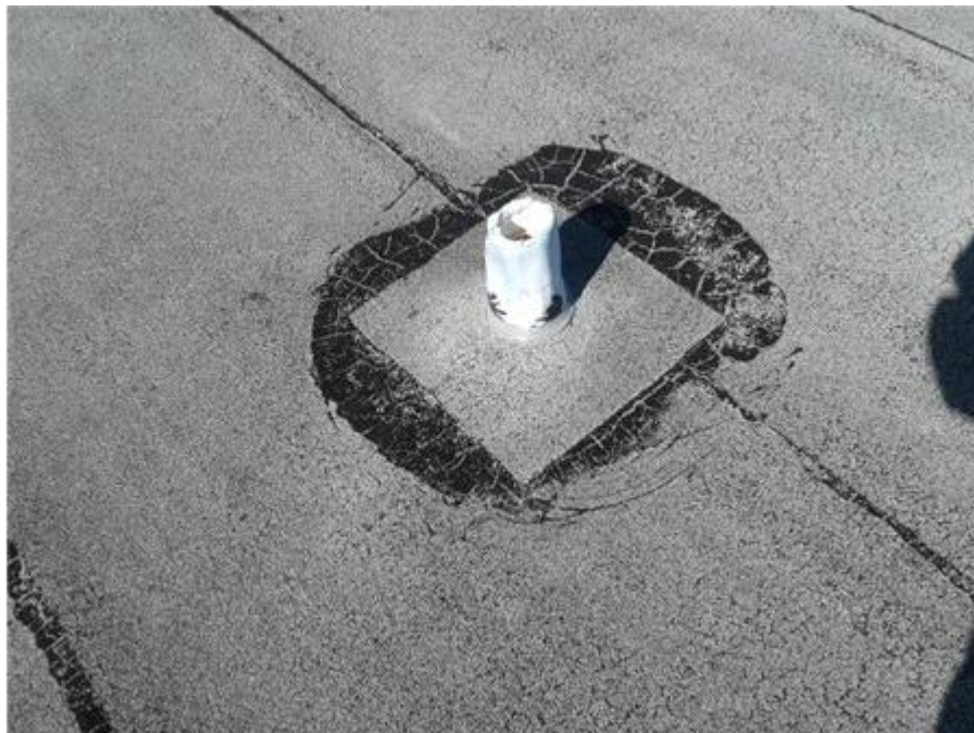
Elevator Shaft Roof: Lead Boots
