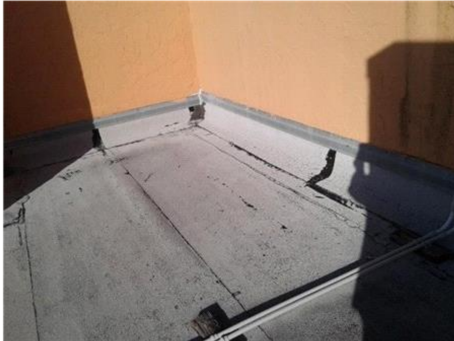
Main Roof: Base Flashings
