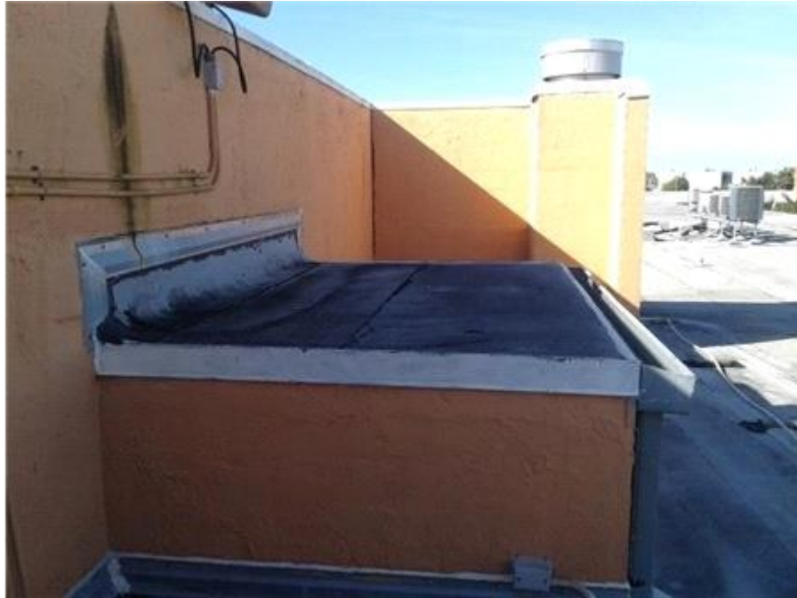
Stairwell Roof: Membrane Overview
