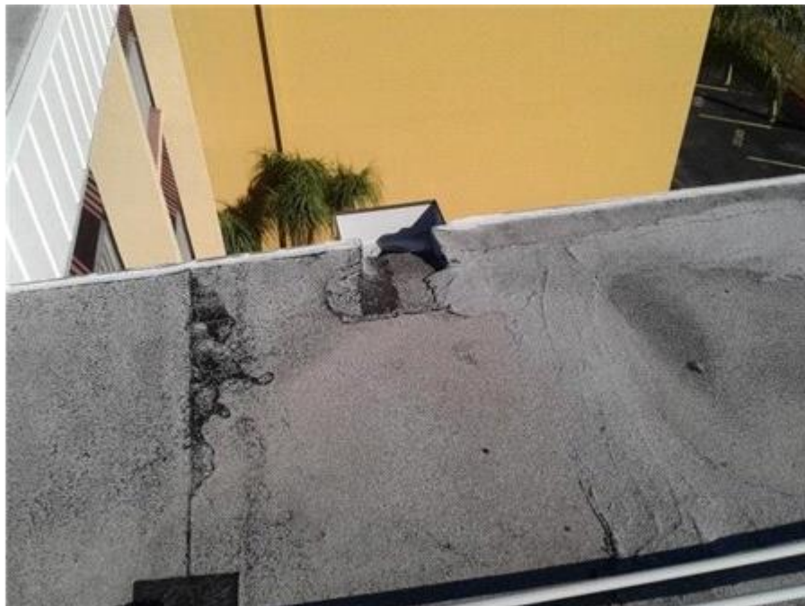
Stairwell Roof: Scuppers
