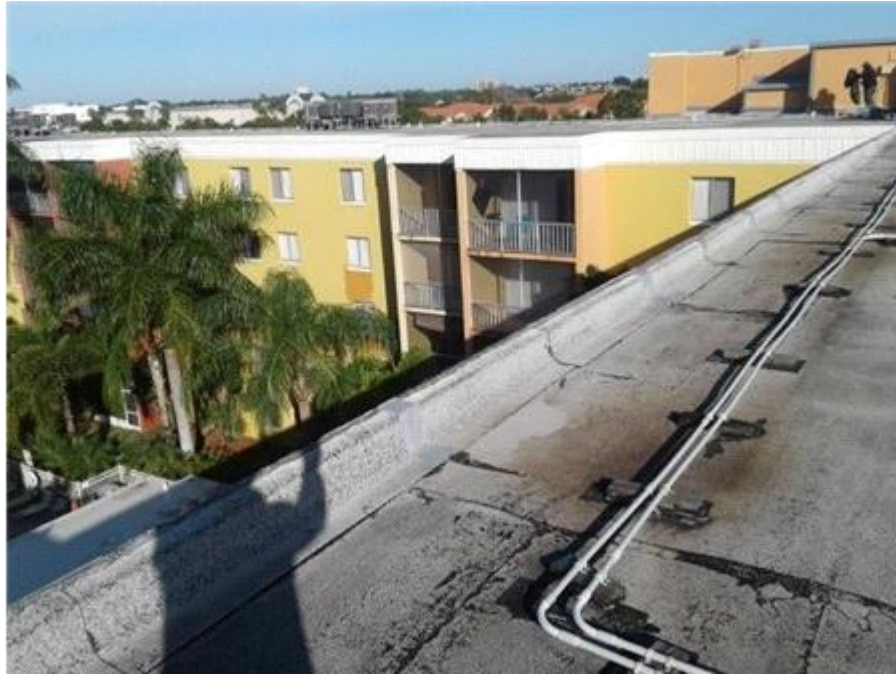
Main Roof: Wall Flashing
