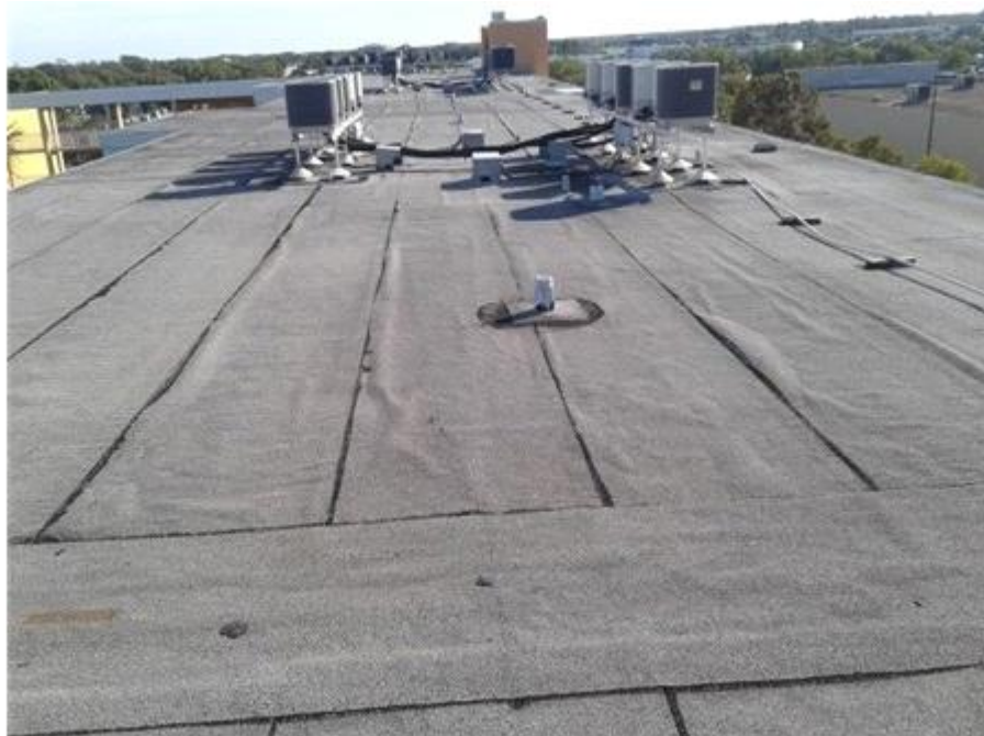
Main Roof: Roof Overview
