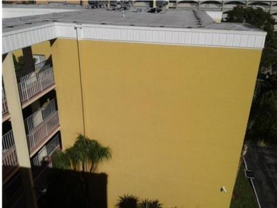
Stairwell Roof: Downspouts
