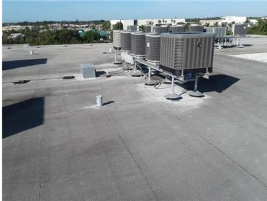
Main Roof: Appearance Overview
