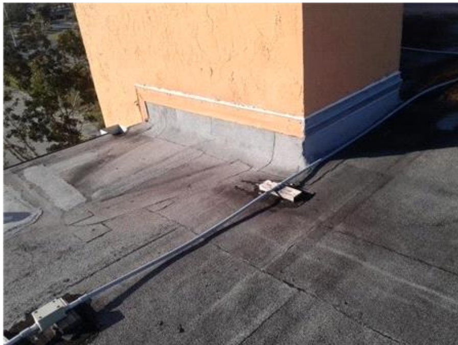
Main Roof: Base Flashings
