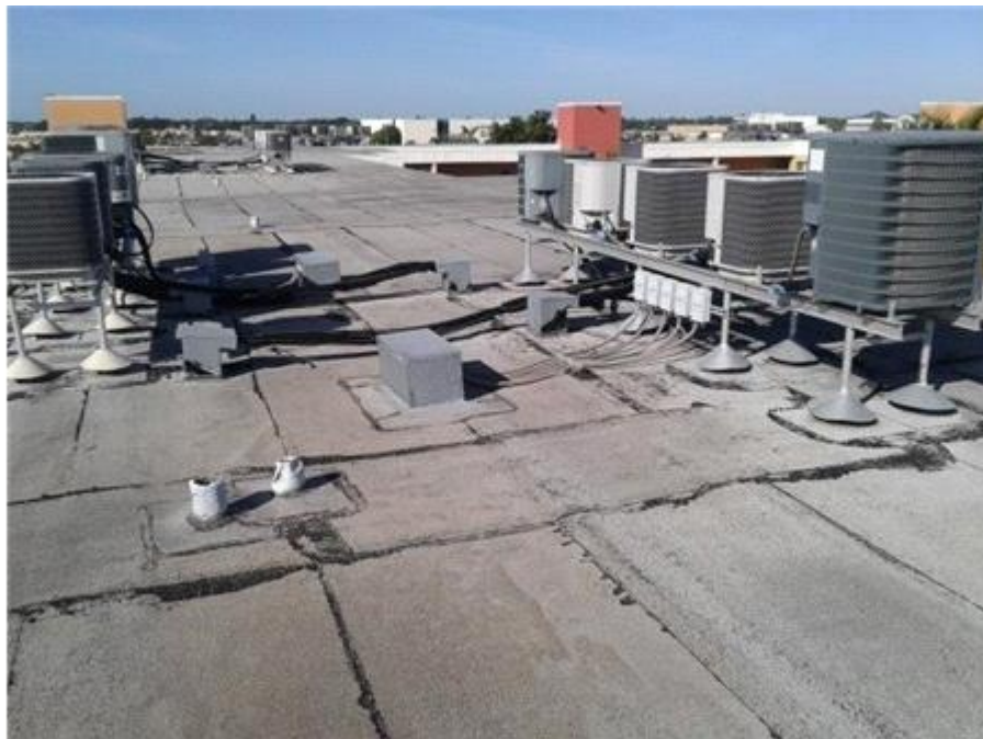
Main Roof: Appearance Overview
