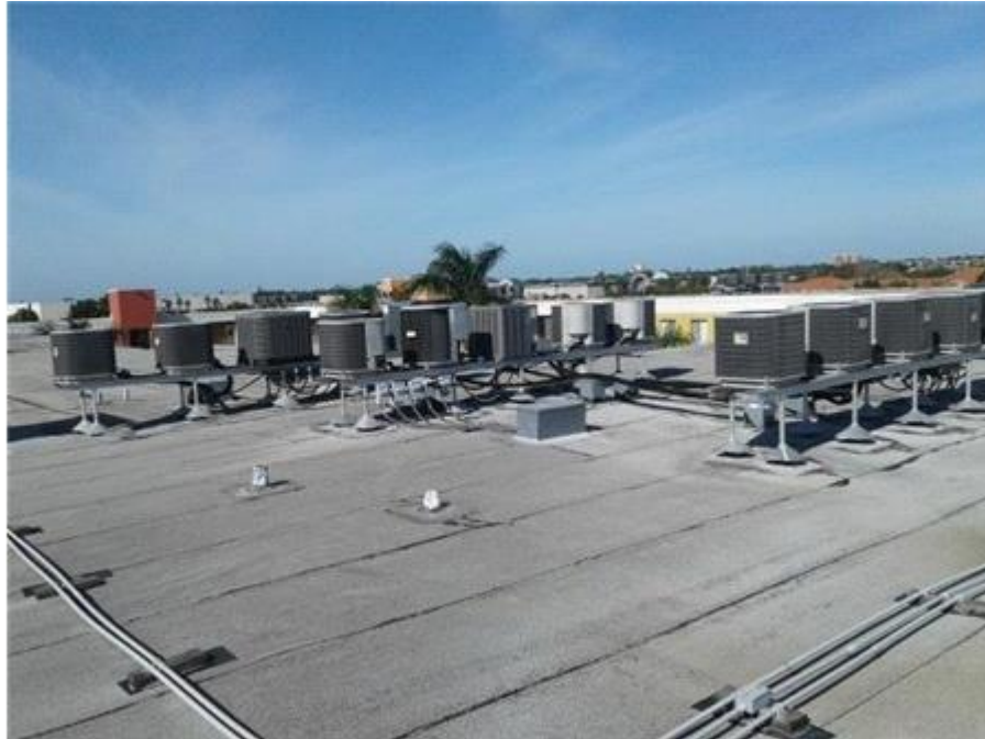
Elevator Shaft Roof: Roof Overview
