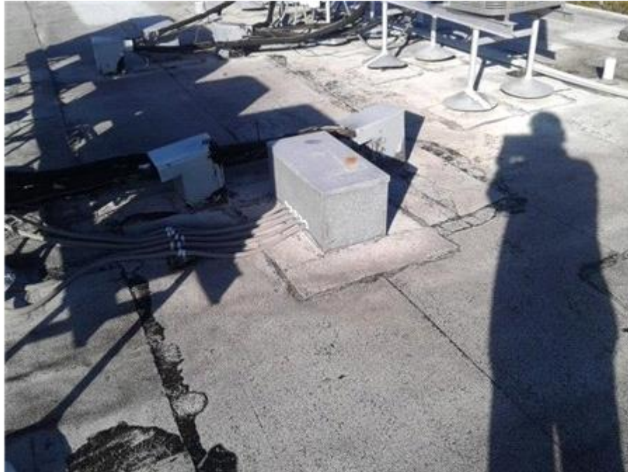
Main Roof: Equipment Housing
