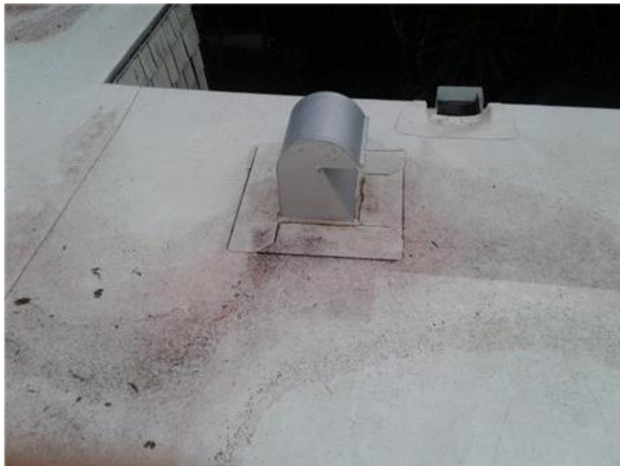
Clubhouse: Roof Vents
