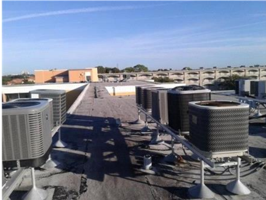
Main Roof: Roof Overview
