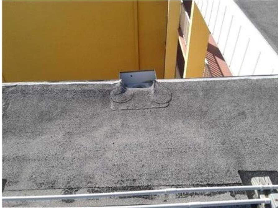
Stairwell Roof: Scuppers
