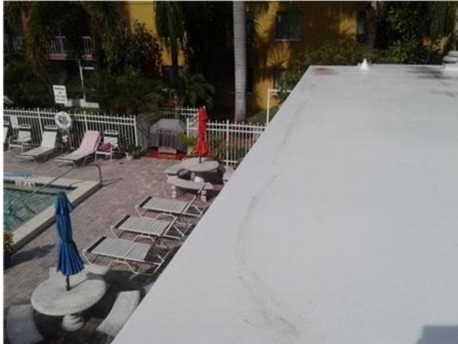
Clubhouse: Roof Edge
