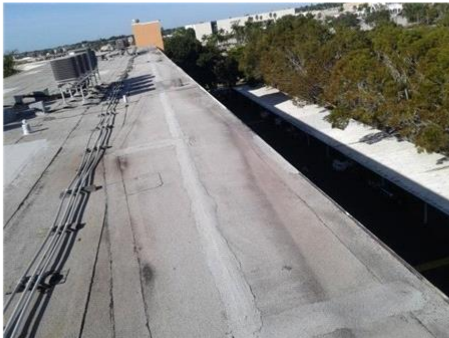
Main Roof: Roof Edge
