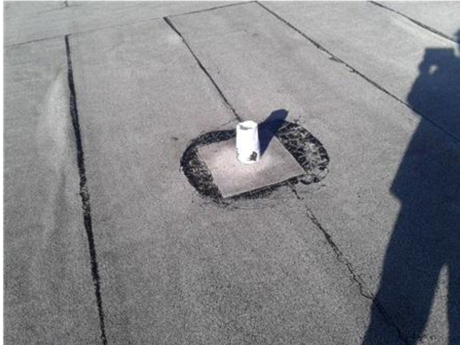
Main Roof: Lead Boots
