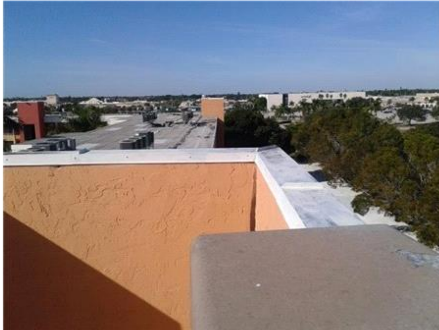
Stairwell Roof: Coping
