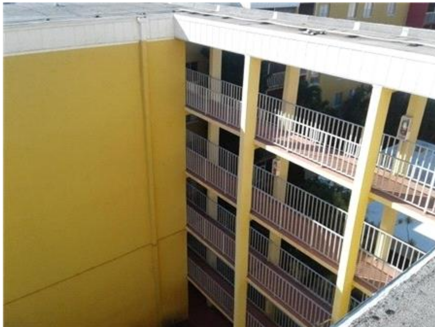
Stairwell Roof: Downspouts
