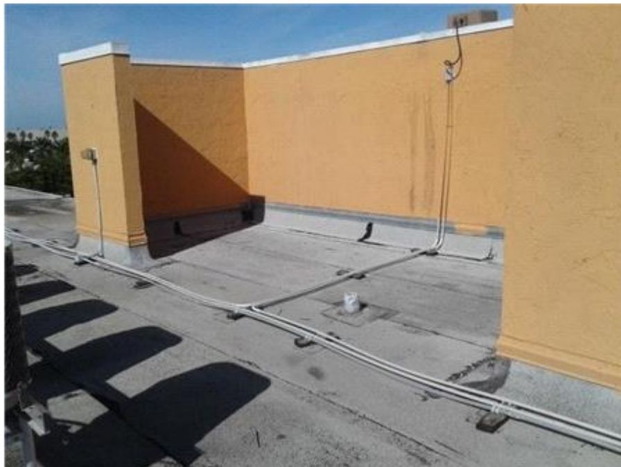
Stairwell Roof: Appearance Overview
