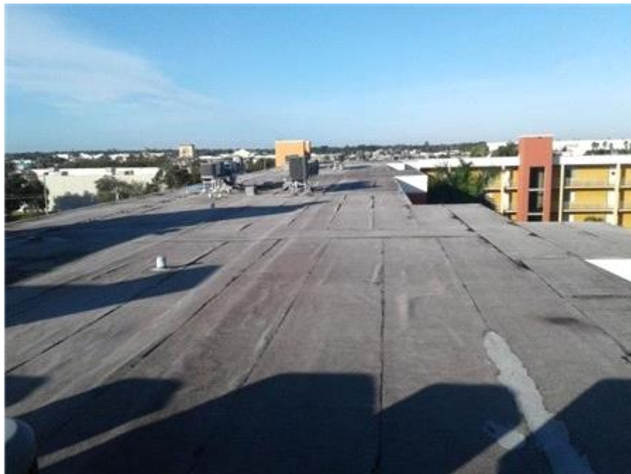
Main Roof: Roof Overview
