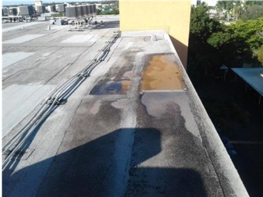
Main Roof: Roof Edge
